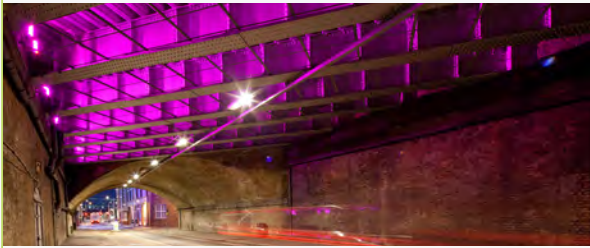
Bermondsey Street tunnel
