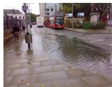
Tooley Street flooding
