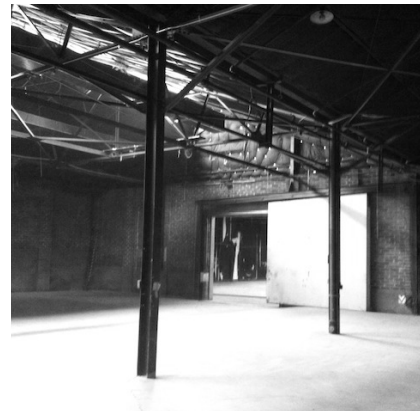
Krog Street Sheet Metal Warehouse
