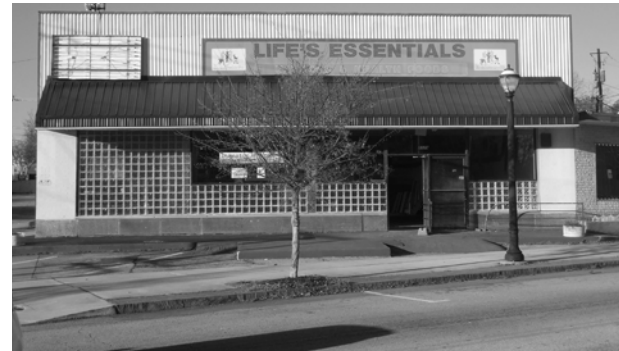
Vacant Grocery Store, 2329 Cascade Road
