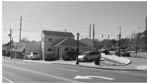
Existing intersection of Cascade Road and Benjamin E. Mays Drive.
