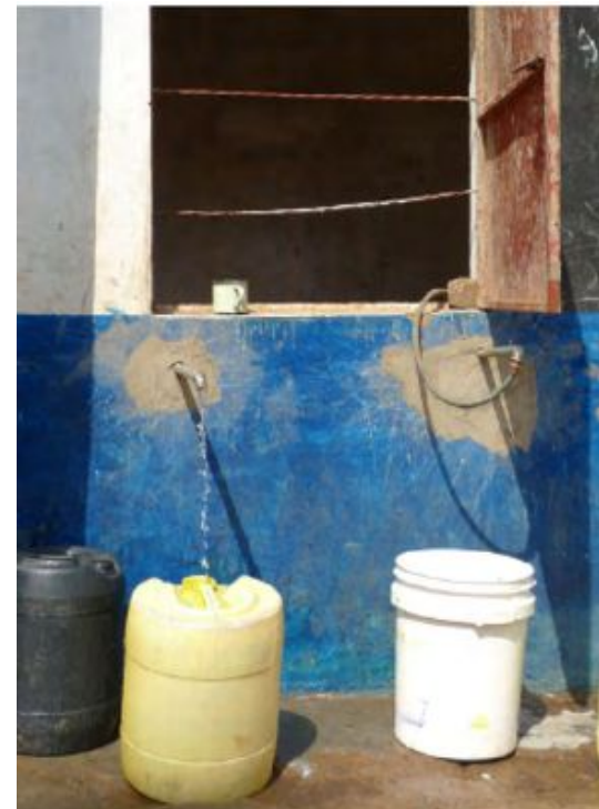
Above: random exposed water pipes, frequently contaminated by sewage Left: typical yard tap
