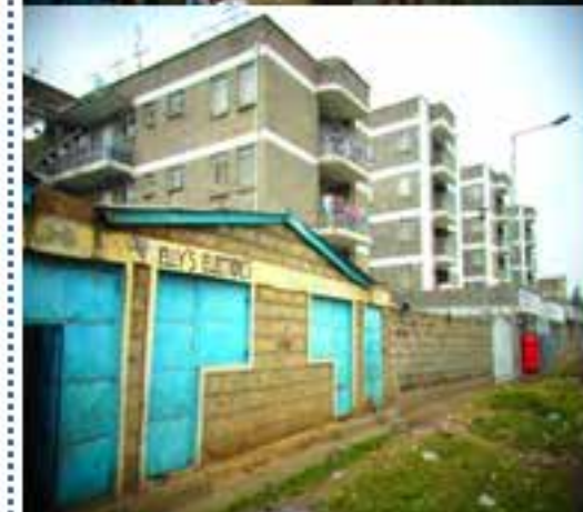
Figure 16. High-rise structures in Motomoto
