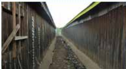
Figure 13. Wood structures in Zone 48 © Z.G.Blanco, CURI 2012
