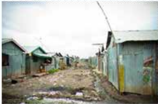
Figure 11. One floor Mabati structures. Riara
