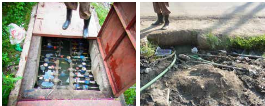
Figure 19(left) Chamber with meters in Riara. Figure 20. (right) Water illegally tapped in Emba-villa.
