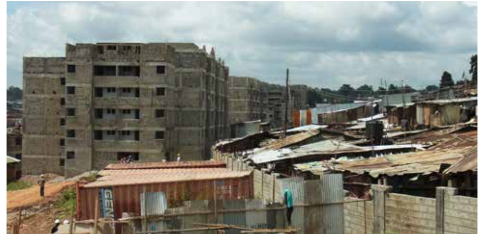
Figure 03. Kibera KENSUP. Soweto A under construction. ©Z.G.Blanco, CURI 2013
