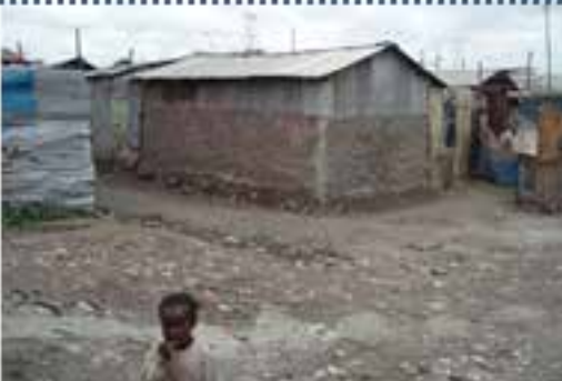
Figure 15. Stone, mud & metallic net tech- nique. © Z.G.Blanco , CURI2012
