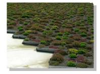
Loose-laid/ built-up: each component of the system is installed separately and they are layered on top of each other.
