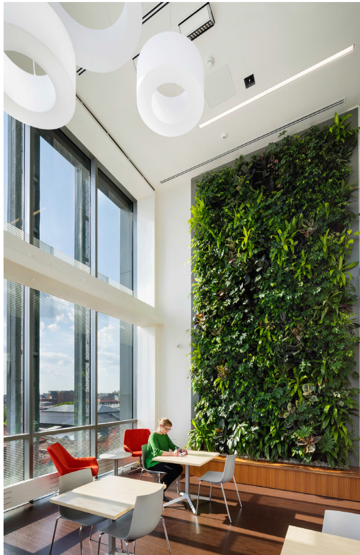
The HVAC-integrated living wall at Weiser Hall at the University of Michigan improves air quality and reduces energy costs. 2018 Award Winner: Diamond Schmitt Architects & Nedlaw Living Walls.
