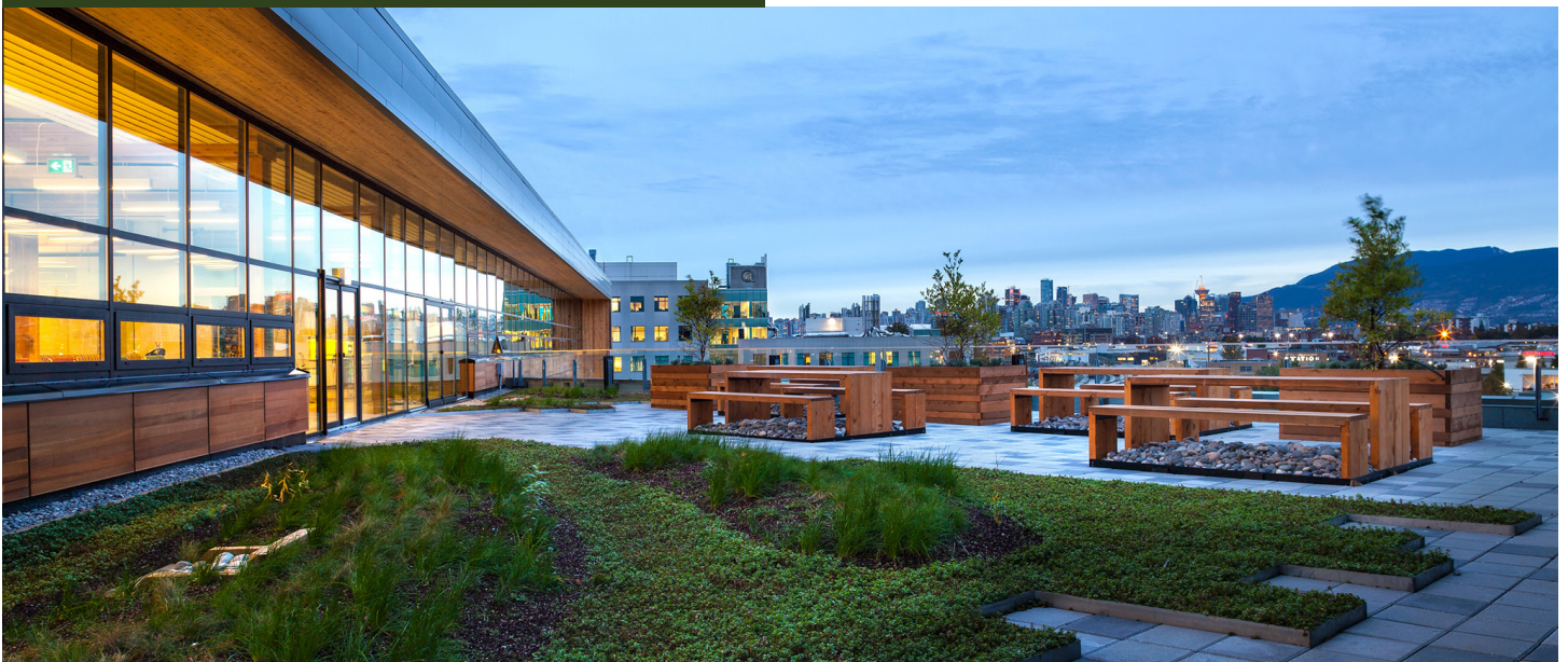
The MEC HQ green roof captures and re-uses rainwater, uses food producing plants, provides amenity space, and features a panoramic view of Vancouver's North Shore Mountains. 2017 Award Winner: Connect Landscape Architecture, Inc.
