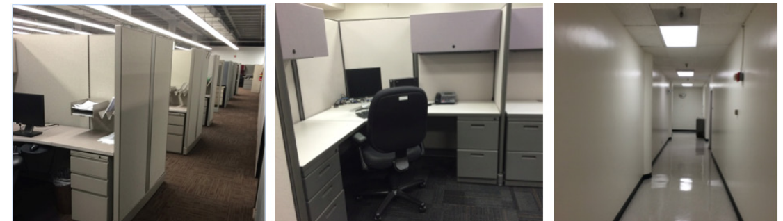
Figure 1: LA County Department of Public Health, IT Offices and Corridors Source: Authors
