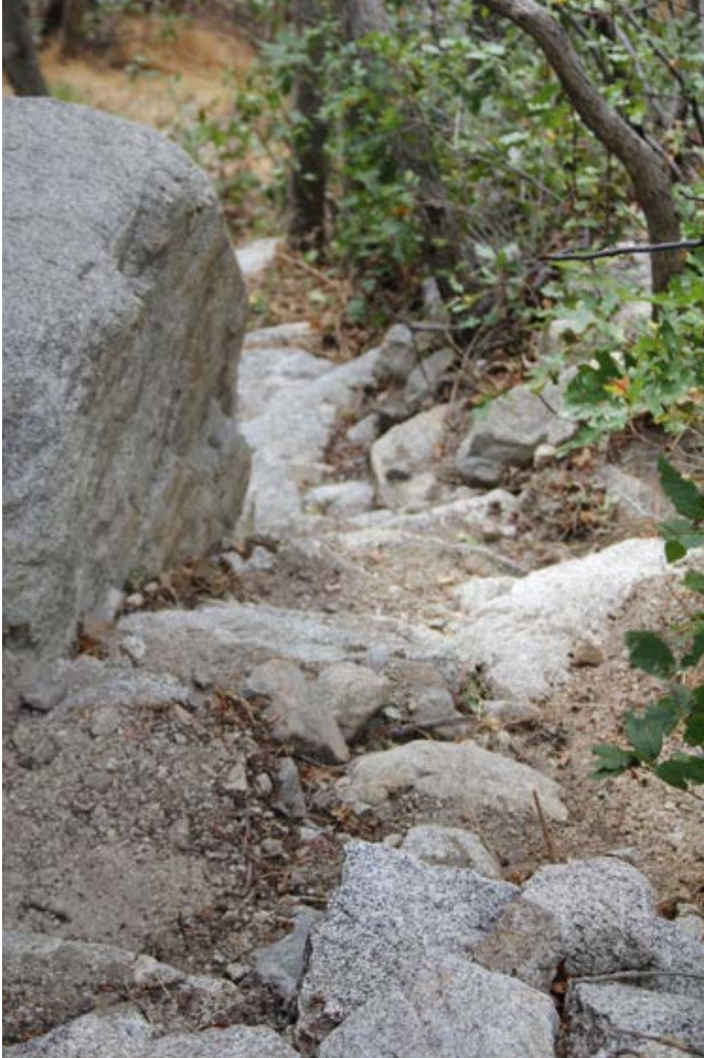
Photograph 10. View of upper trail that leads to Memorial Day Buttress showing condition of recent trail work. Camera view northwest.
