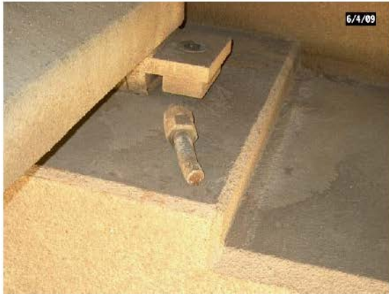
Figure 89. 19 th Street/I-35 Bridge sheared anchor bolts in 2009
