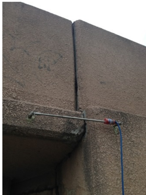
Figure 43. East abutment of SH-3 north bridge over BNSF railroad – CMA2 crackmeter
