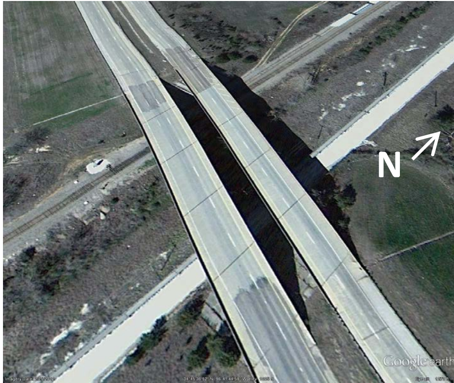
Figure 34. SH-3 bridges over BNSF railroad
