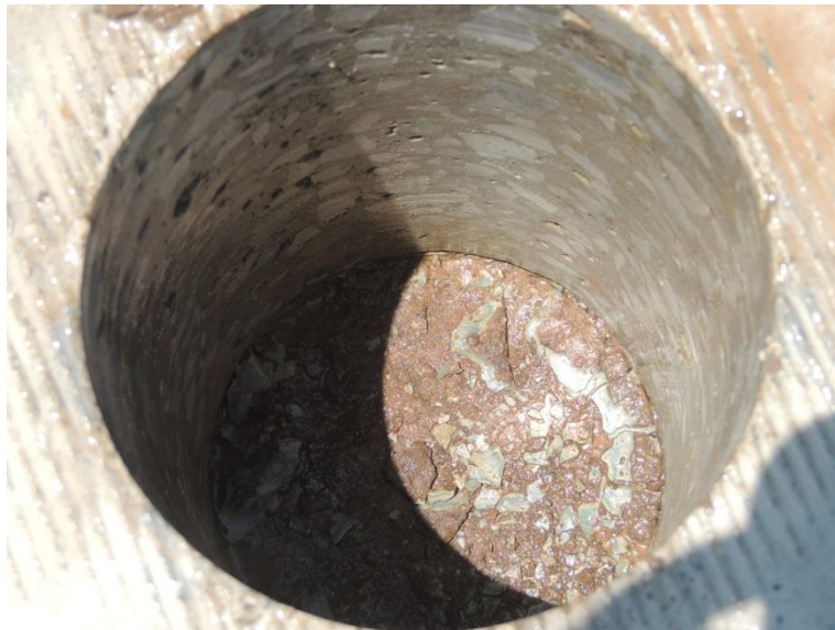
Figure 10. Picture of De-bonding.
