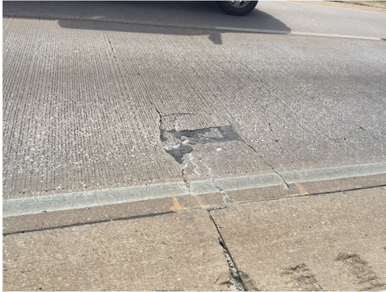
Figure 14. Picture of a Typical Punchout from I-35 SB.
