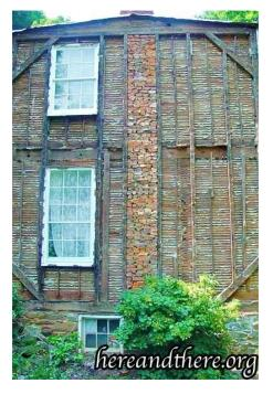
Construction Era: Knowledge of building eras can indicate the building materials, special hazards, fire behavior, floor layout and structural integrity under fire conditions. Structures built prior to the "new" national wood standard (1924) used full dimensional lumber floor joists and tongue and groove (T&G) floor decking. These materials held up considerably longer under fire conditions compared with engineered wood products of the mid 1980s.
