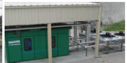
**Air Cooled Condensers for Engine Cooling**
