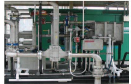
**Gas Piping for Digester, Chiller Glycol Heat Exchanger, Flame Arrestor, Gas Meter, and Gas Pressure Booster**
