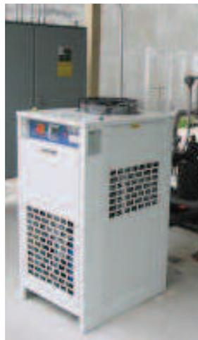
**Air Cooled Chiller System for Gas Conditioning**
