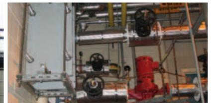
**Heat Exchanger Capturing Heat from Generator for Boiler**
