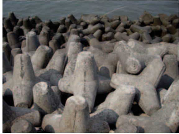
Fig. 431 | Photograph 2014, concrete tetrapods at Marine Parade, Bombay, India.
