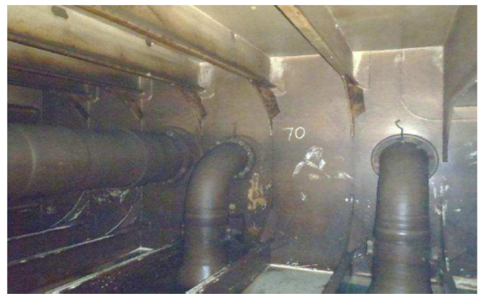
Figure 5: Typical oil tanker double bottom internals, about 2.5 m height
