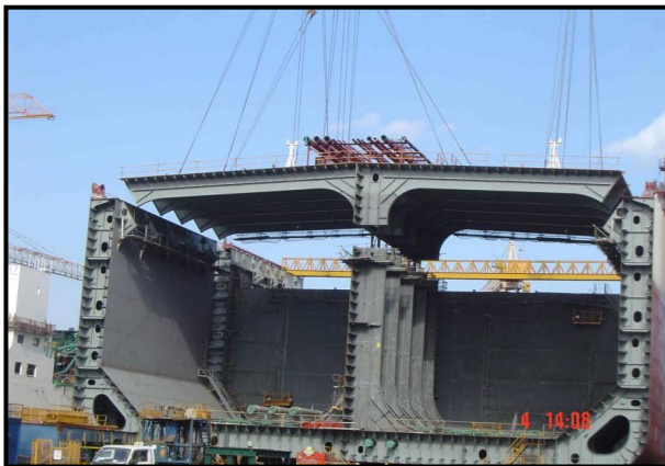
Figure 2: Double hull tanker under construction
