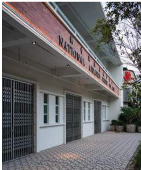
The conserved National Aerated Water Building is a standalone two-storey commercial building, although it sits within the development
