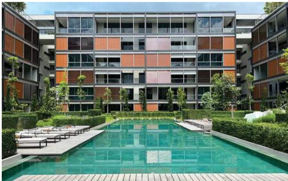
The 30m swimming pool is set centrally along the main axial view of the courtyard
