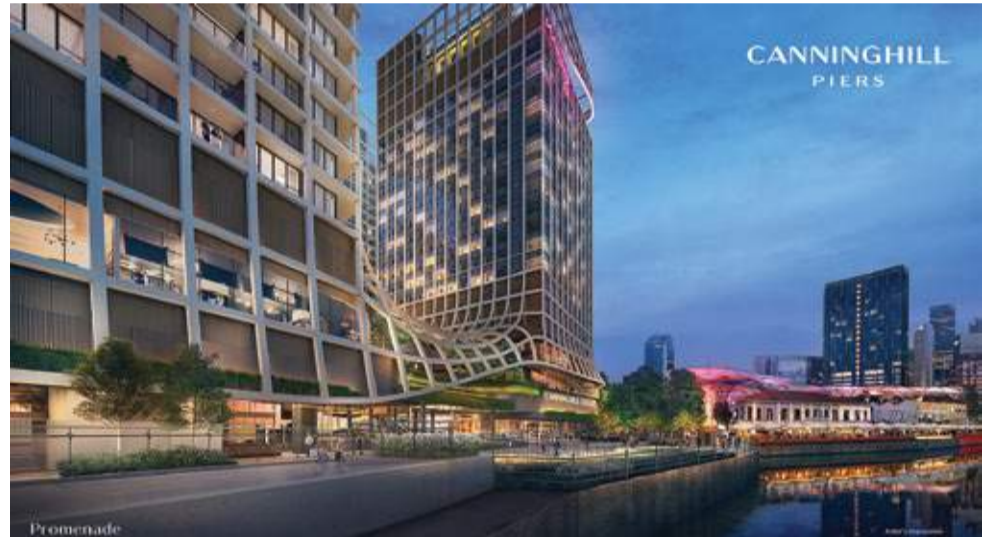
CanningHill Piers hosts a diverse range of civic spaces and a public riverfront promenade
