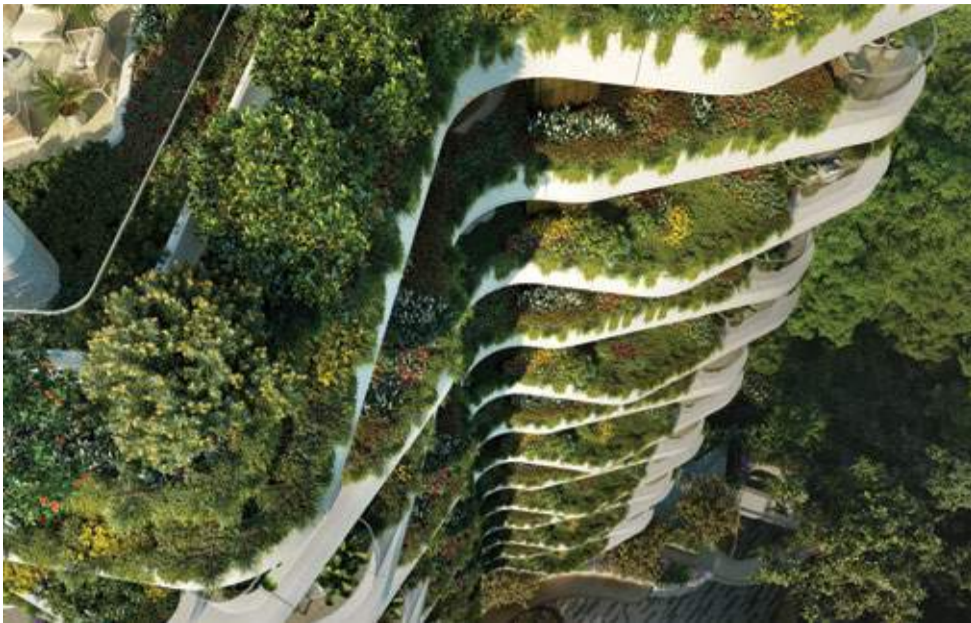
By deploying the strategy of having "undulating overhanging balconies", the living spaces and bedrooms within the apartments are shaded from the heat
