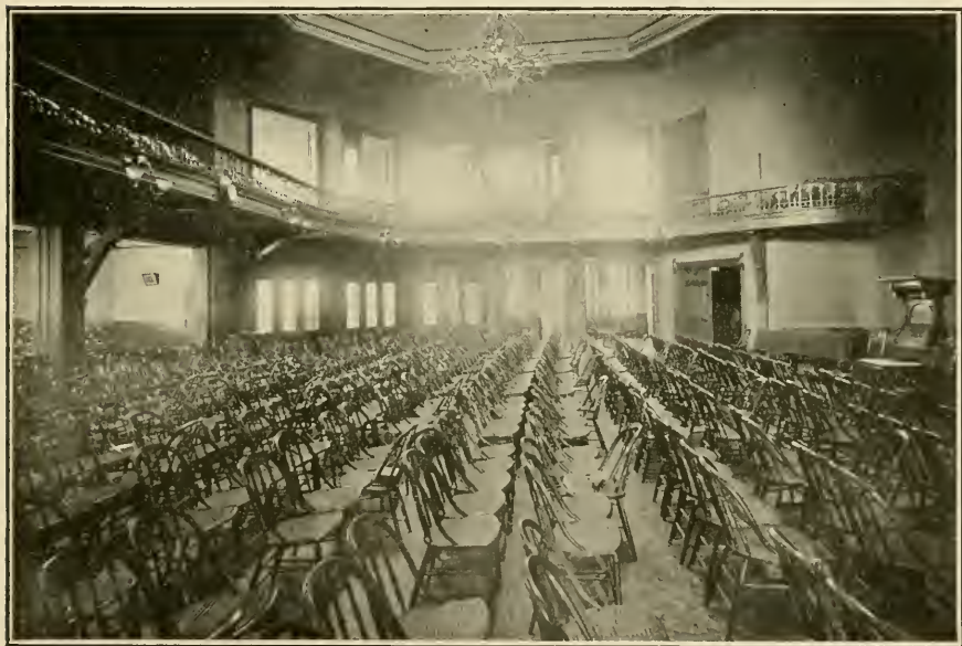
Woodland Avenue Presbyterian Sunday-school Building—Interior.
