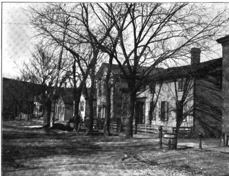
NORTH SIDE OF WEST BROAD ST., BELOIT, JANUARY, 1900.
