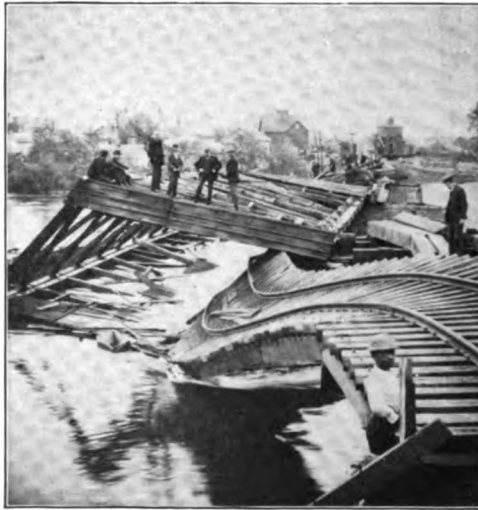
NORTHWESTERN R. R. BRIDGE, BELOIT, WIS. Tornado Ruin, June 12, 1883. Looking S. E
