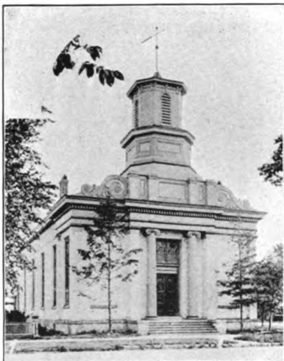
STEEPLE REBUILT AFTER TORNADO.
