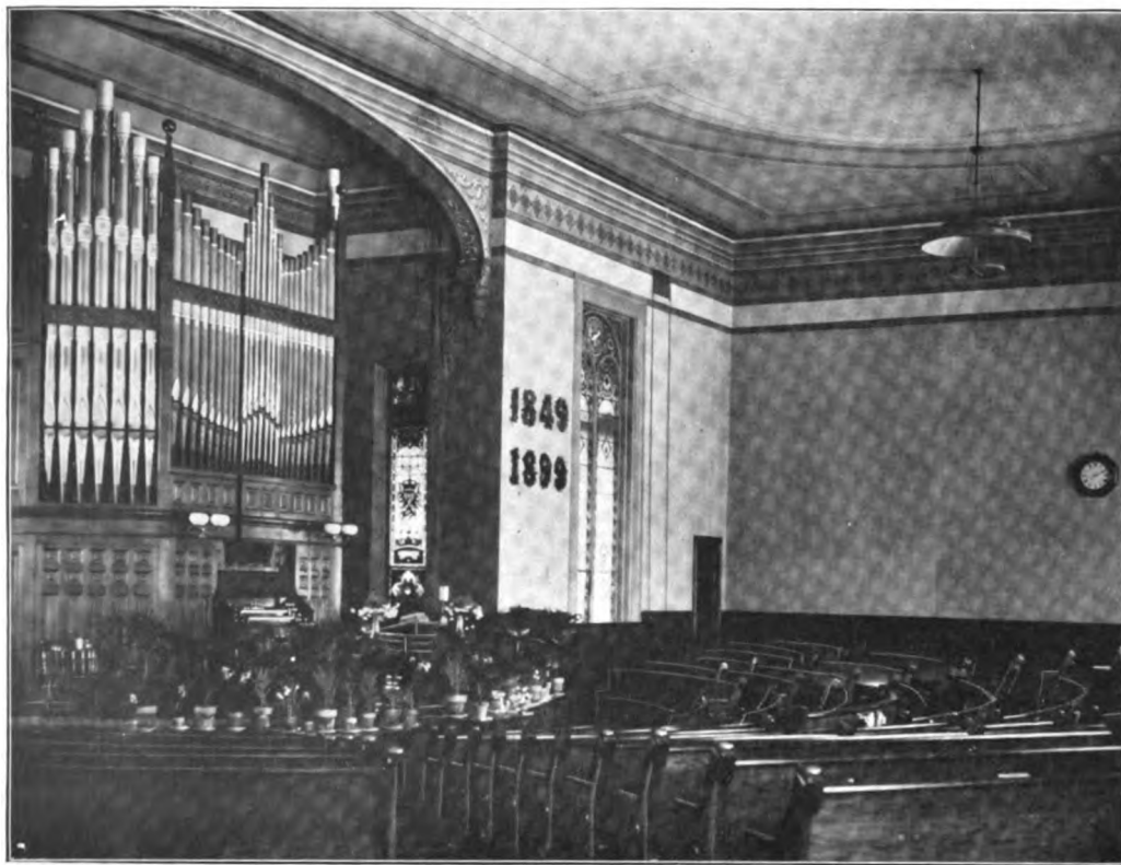
INTERIOR FIRST PRESBYTERIAN CHURCH.
