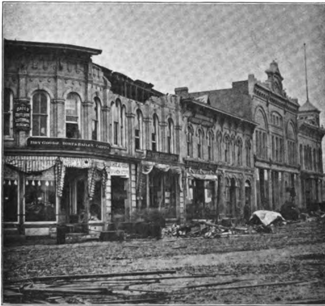
SOUTH SIDE OF EAST BRIDGE ST., BELOIT, WIS. After the Tornado of June 11, 1883.
