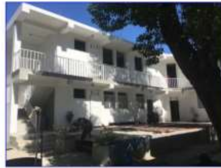
The Radia Laboratory of Science and Technology exemplifies The Haitian Project's commitment to environmental stewardship; it is fully solar powered and is the first building on the LCS Santo 5 campus to incorporate steel elements to reduce the amount of concrete in construction.
