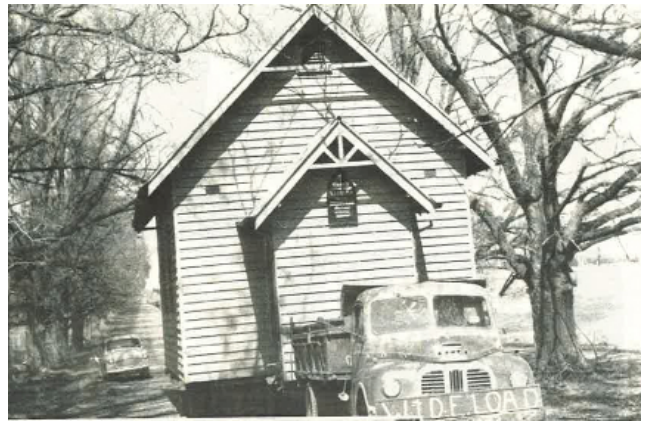
The original building being moved to the university church land
