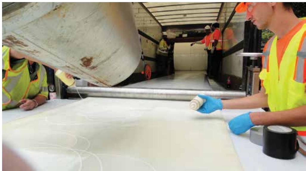
Liner wet out involves mixing two-part chemicals
