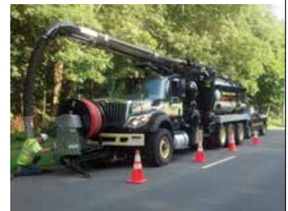
Sewer Cleaning and TV Inspection
