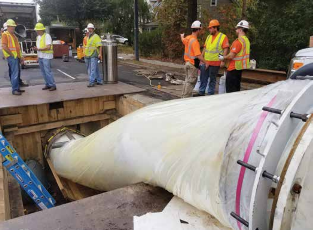
Liner entering host pipe after going through inversion cone
