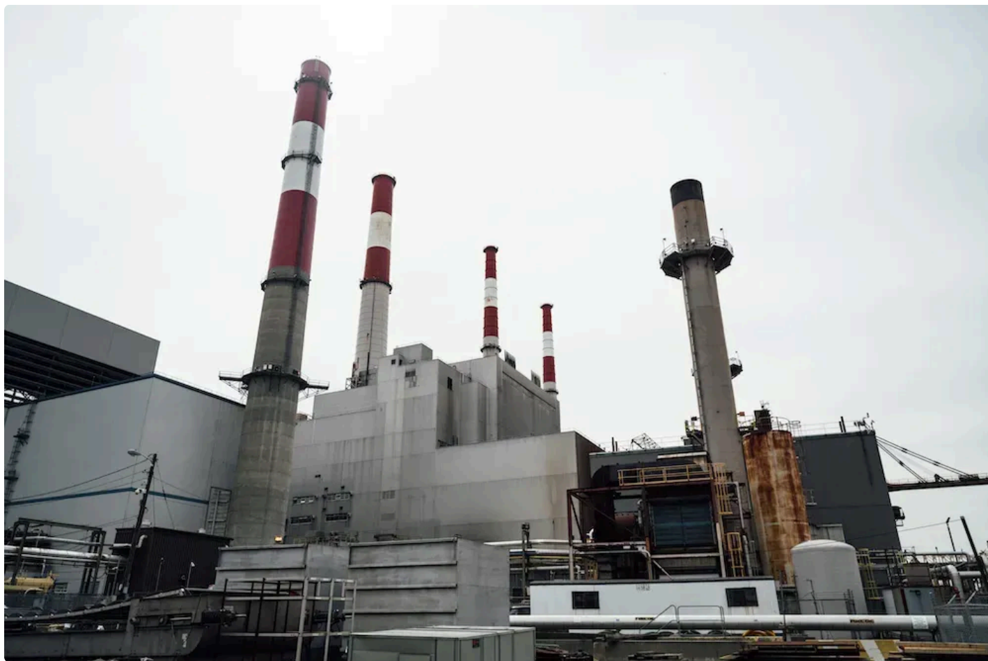
The Ravenswood Generating Station in Queens. (Scott Heins / Hell Gate)
