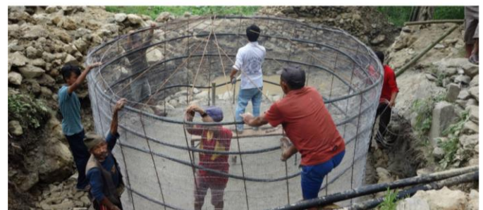
Figure 7. Constructing a new rainwater tank in Sandikohla, 2013
