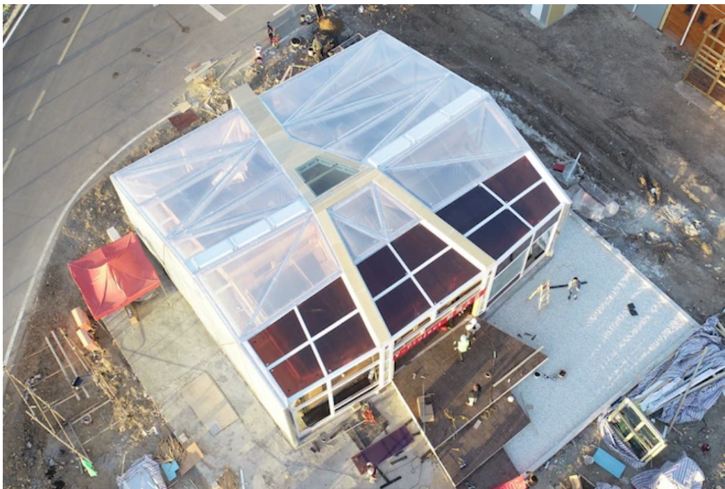
Figure 13b - Aerial photo of the completed SDC Y-House on site
