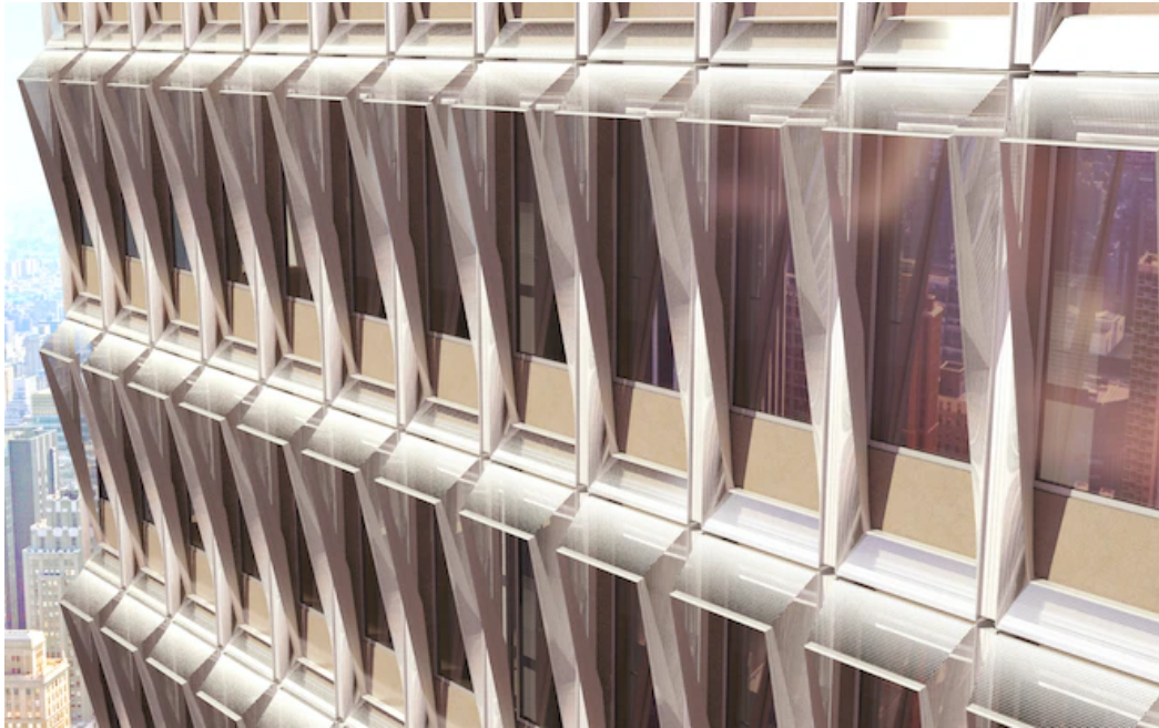
Figure 20 - Overall image of the Thermalswitch unit installed (summer orientation)
