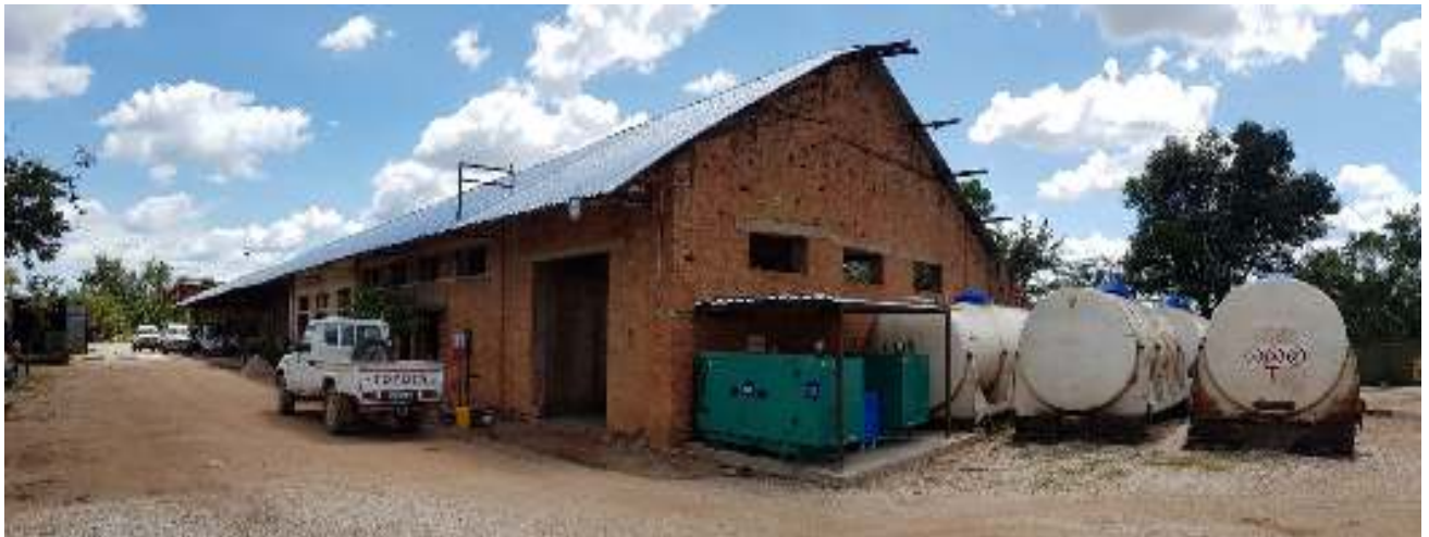
Refurbished Core yard and logging facilities including diesel storage tanks (100,000lts capacity)
