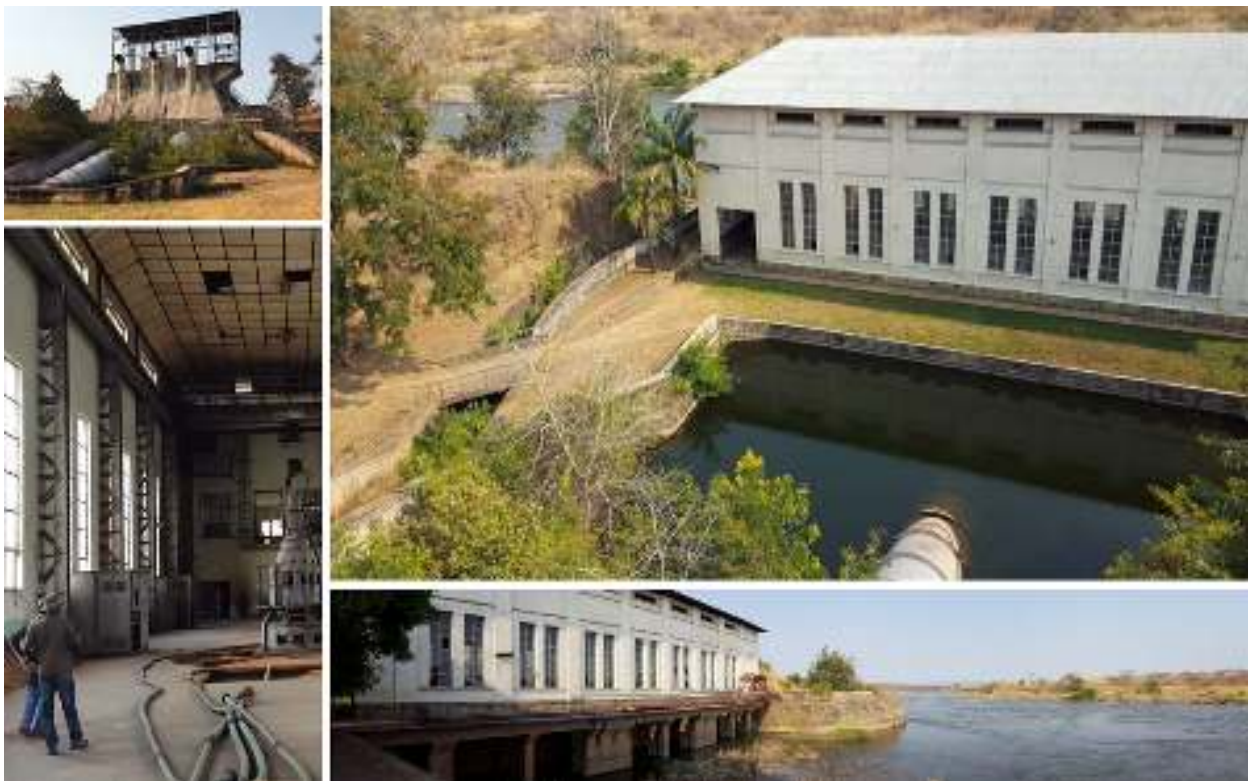
Images of the Piana Mwanga 32Mw Hydro Facility
