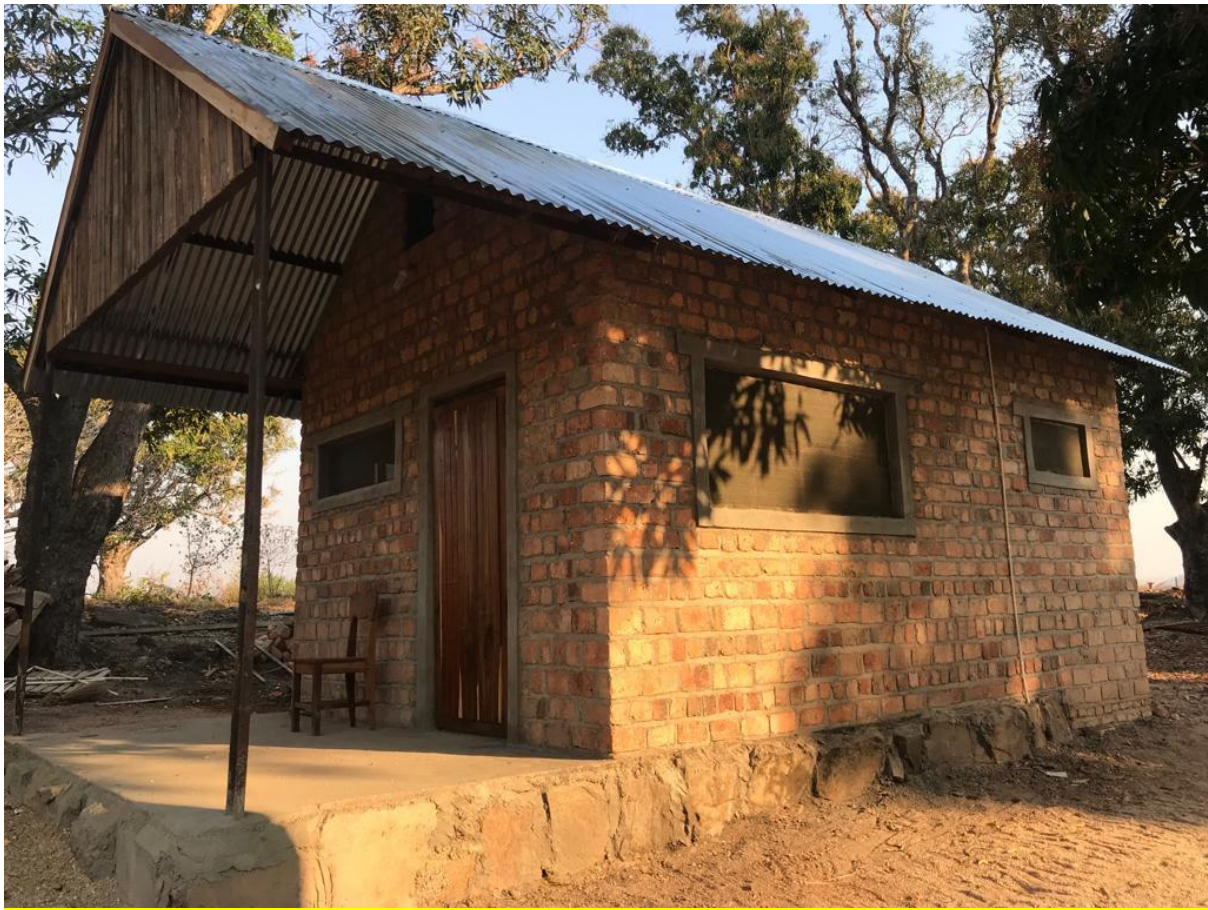
Figure 15: Single-man accommodation quarters at Camp Colline
