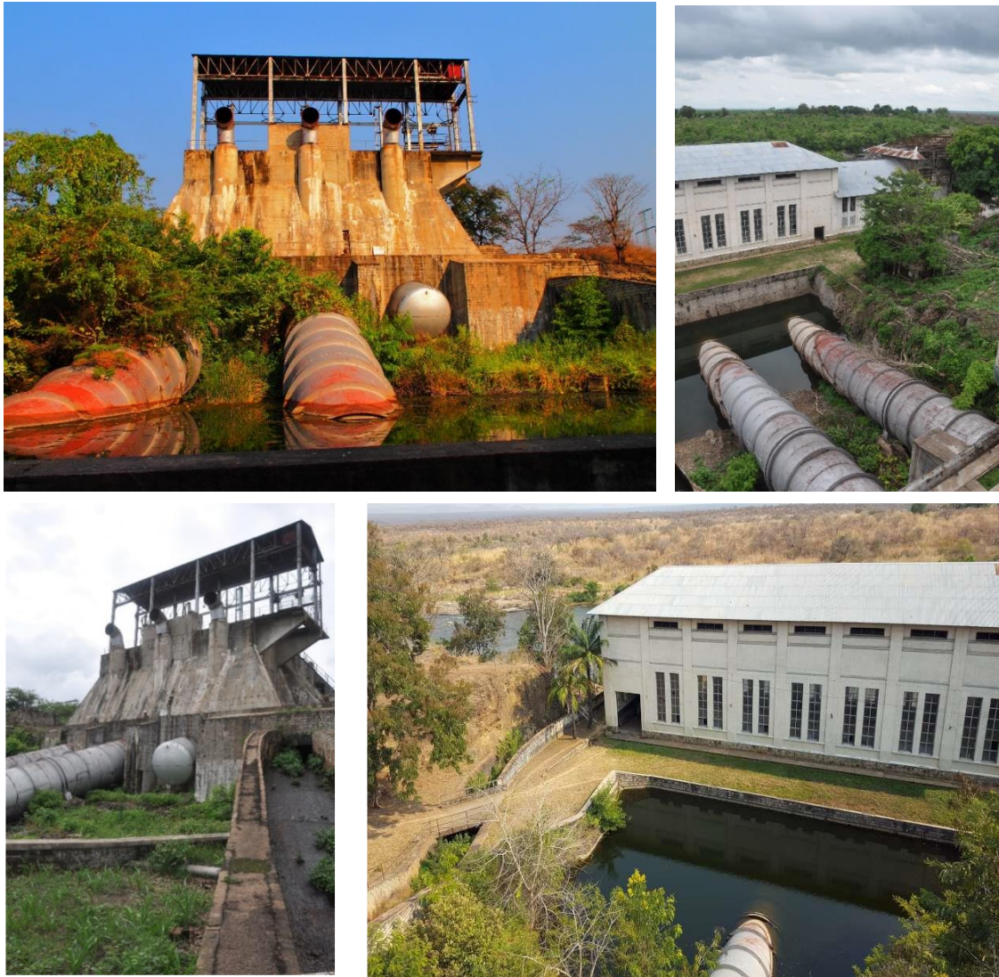
Figures 6-9: The Mpiana Mwanga Hydro Electric Power Plant on the Luvua River
