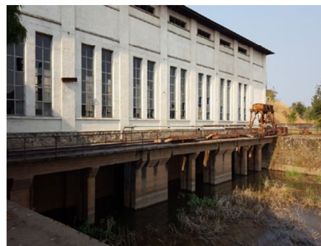
Figures 6-9: The Mpiana Mwanga Hydro Electric Power Plant on the Luvua River
