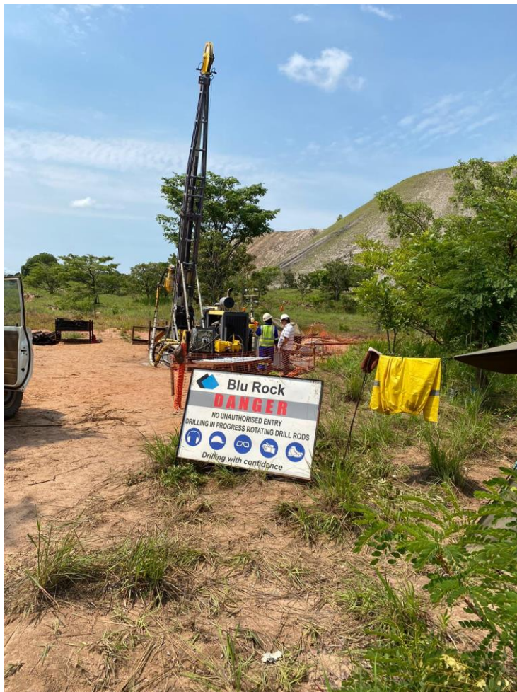
Figure 5: Drill rig at drillhole MO22DD028
