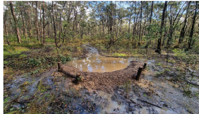
21 ponds along Peters Gully creekline to catch water in high rainfall periods, slowing down water flow for gully hydration.
