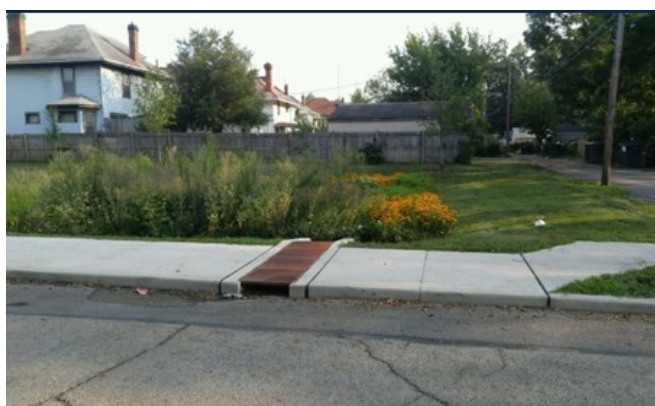
A rain garden completed through the Blueprint Columbus program at 842 Gilbert Street
