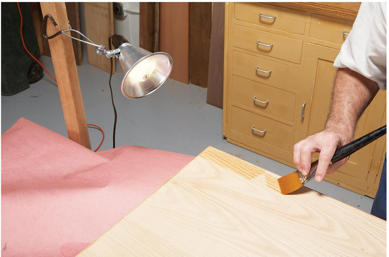
*Set up a light source at a low angle so it rakes the work area. A raking light will show defects like drips and "holidays" (places you missed) before it's too late to correct them.*
