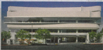
ABOVE + INSET As the first phase of the master plan for West Hollywood Park, the newly designed public library meets the city's goals for a larger, state-of-the-art facility and increased open park space.
