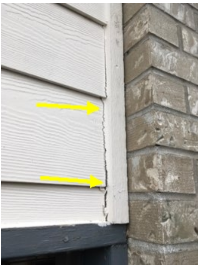
Splitting caulking above garage.
