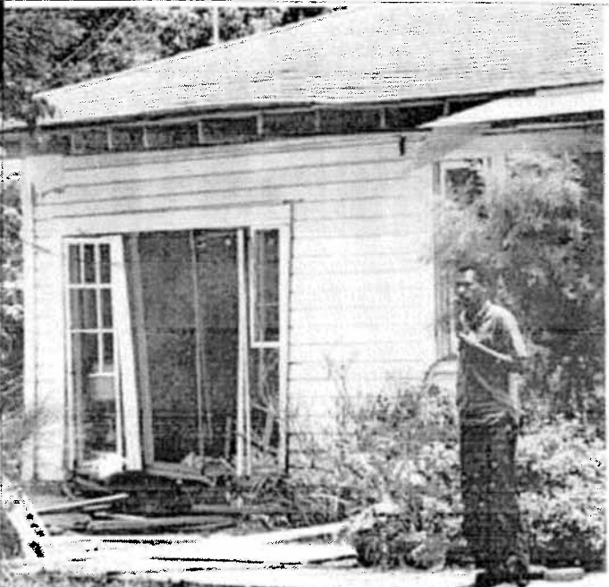
SNCC WORKER JESSE HARRIS surveys damage of SNCC FREEDOM HOUSE in McComb, Miss. A SNCC worker and summer volunteer were injured.
