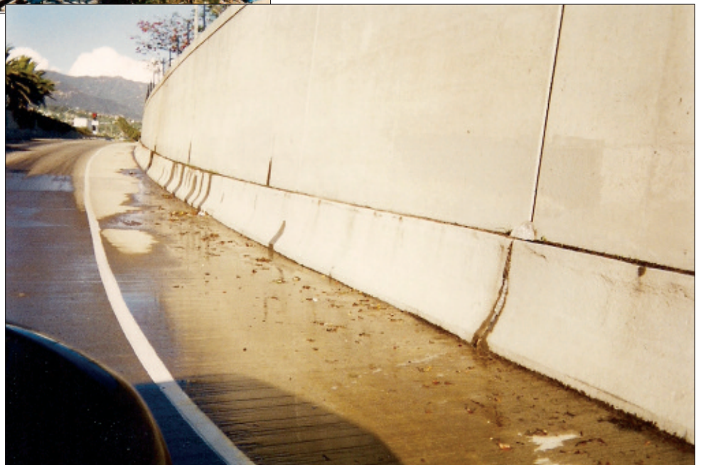
The leaking wall at Garden Street 101 onramp South
