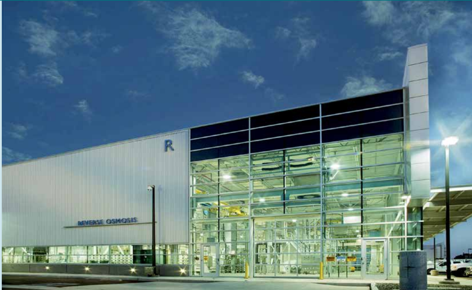
A sample of our vision for advanced water recycling: the Reverse Osmosis facility from Orange County's Groundwater Replenishment System. (Photo Credit: Larny Mack, Courtesy of CDM)
