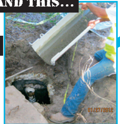
Abandoning old septic system at Sand Point
