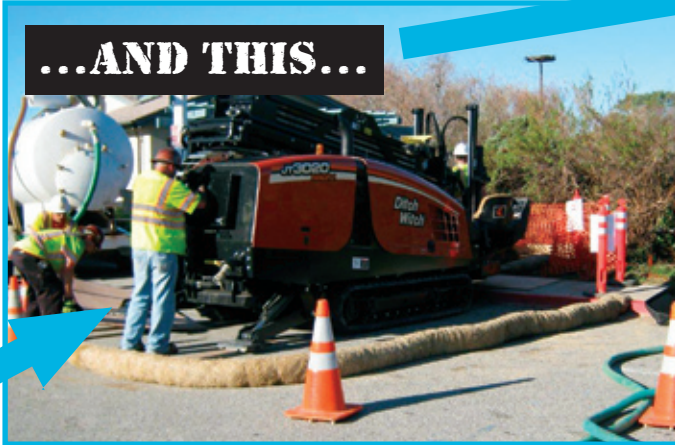
Setting up at Sandyland, to abandon septic systems, connect to sewer.
