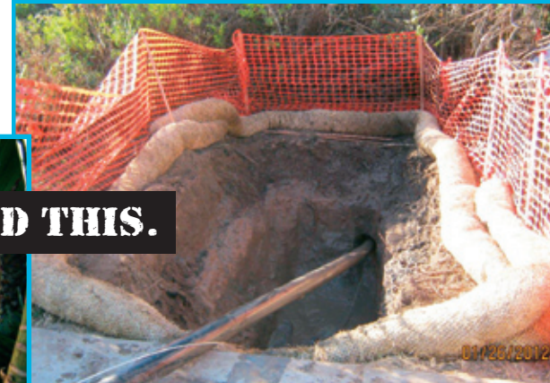
Inserting 3" pipe into old septic system hole at Sandyland.
