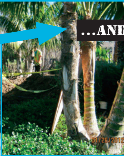
Locating septic system at Sandyland...
