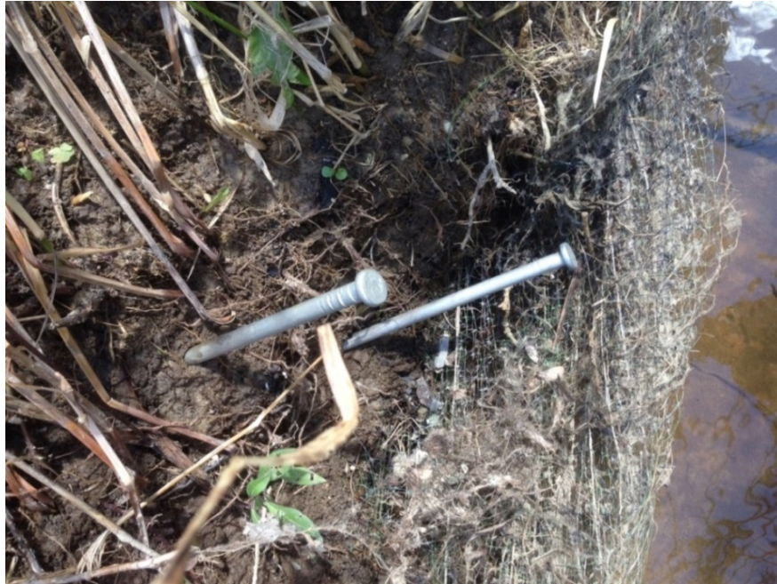
Figure 20. Exposed erosion pins at Station 3.
