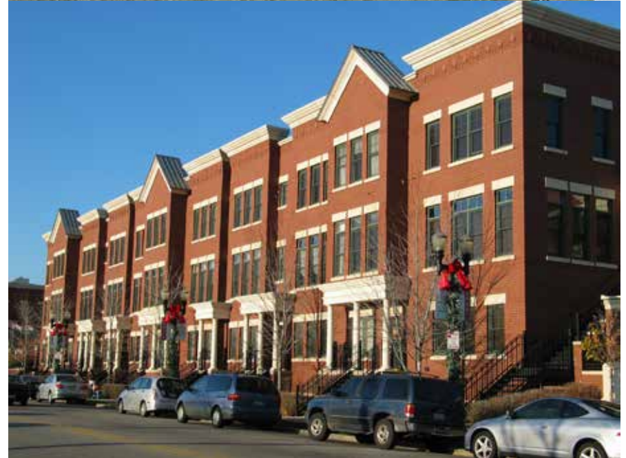
EXAMPLES OF ROWHOUSES WITH HIGH QUALITY EXTERIOR FINISH MATERIALS
