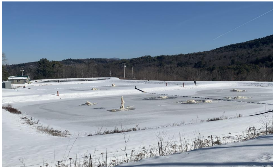
“The New Aeration System is Completed”
