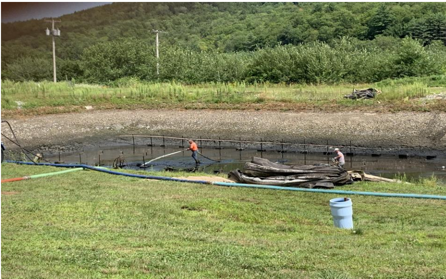
“Cleaning the Lagoons at the Cavendish Treatment Plant”
