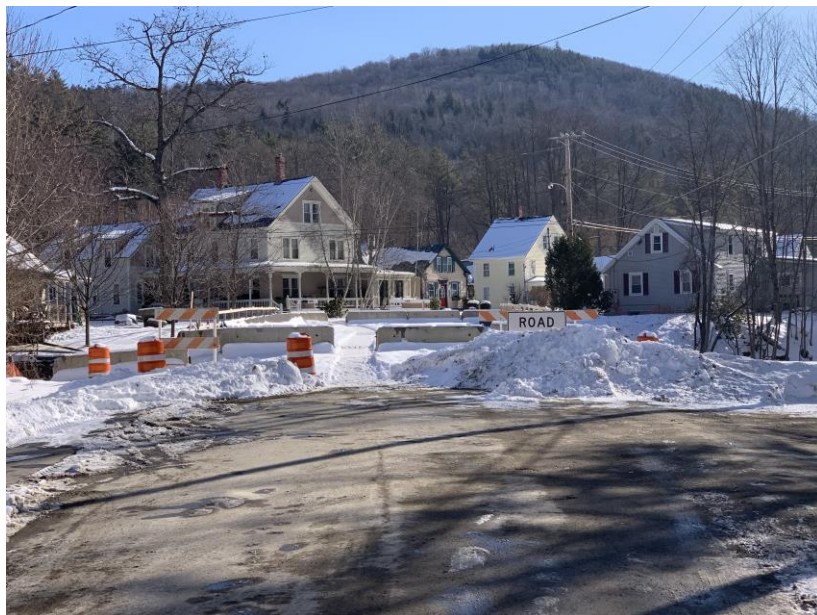
Depot Street Bridge Under Construction
