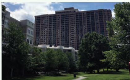
The Skyline neighborhood of Fairfax County includes several large-scale apartment and condominium towers.
