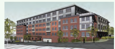
Wesley Housing Development Corporation intends to acquire and redevelop a 12-unit Fairfax County property near the Huntington WMATA Station into two mixed-use buildings with 126 affordable units (rendering above). This effort was made possible by zoning/land use changes and will require the use of local and state capital sources.
