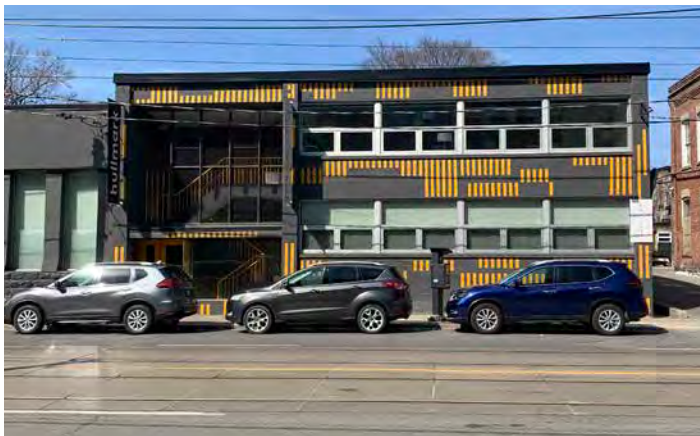
East elevation of 342 Dufferin Street along Dufferin Street.
