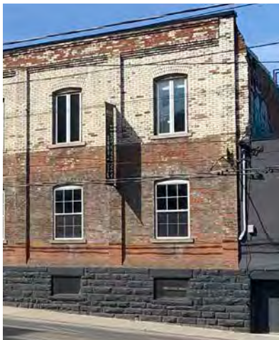
Rusticated stone base and sills. Buff brick sills. Corbelling. Red brick materiality.
