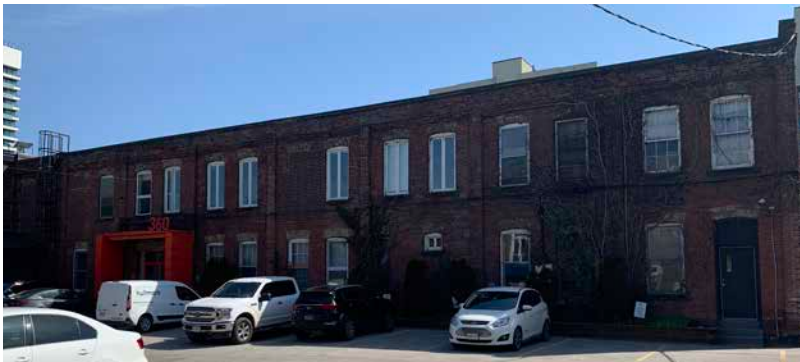
West elevation of 360 Dufferin Street from interior courtyard parking area.
