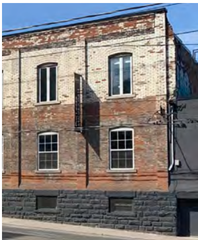
Rusticated stone base and sills. Buff brick sills. Corbelling. Red brick materiality.
