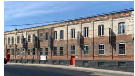
East elevation of 360 Dufferin Street along Dufferin Street.
