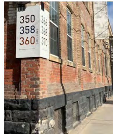
360 Dufferin Street new signage and corbelling above raised basement windows (ERA, 2021).
