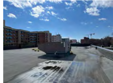
Roof condition (ERA, 2022).
