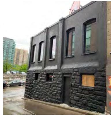
366-370 Dufferin Street north elevation (ERA, 2021).
