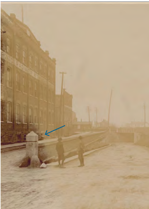
c. 1896-1897 view north on Dufferin Street. The building at 366-370 Dufferin Street is seen on the left, before the basement is excavated and exposed as part of the road regrading project for the rail underpass. (City of Toronto Archives; Annotated by ERA).
