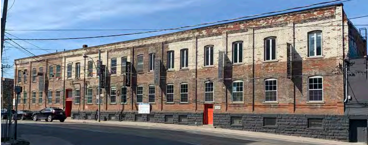
East elevation of 360 Dufferin Street along Dufferin Street.
