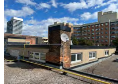
South and west elevation and chimney at 342 Dufferin Street (ERA, 2021).
