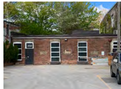
East elevation of 350 Dufferin St. Note: this address is not noted on the property data map (ERA, 2021).
