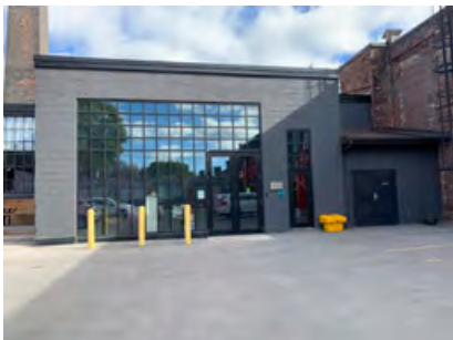
376R Dufferin Street, south elevation (ERA, 2021).
