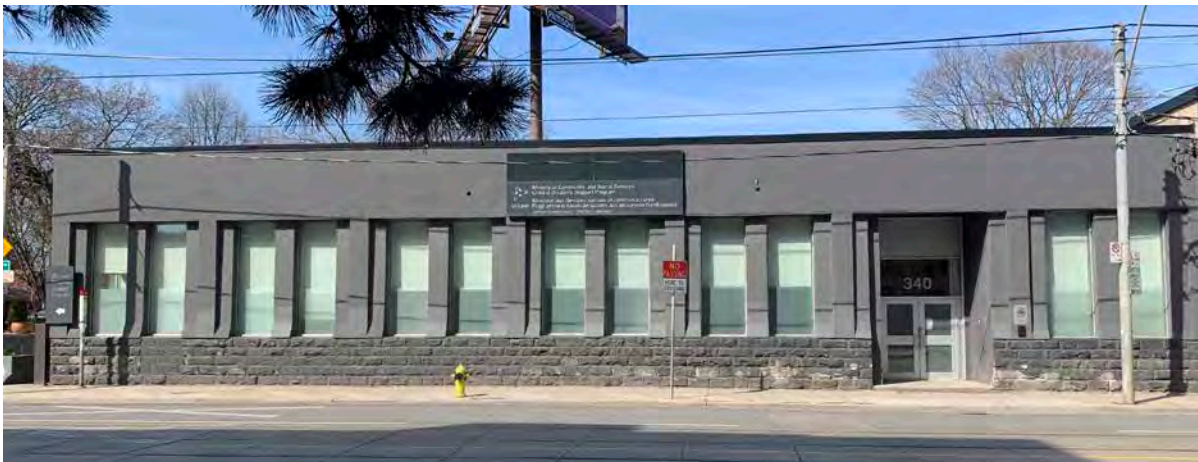
East elevation of 340 Dufferin Street along Dufferin Street.
