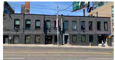
East elevation of 366-370 Dufferin Street along Dufferin Street.
