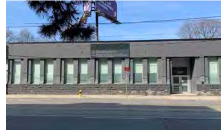
East elevation of 340 Dufferin Street along Dufferin Street.
