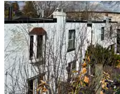
East elevation of 1, 3, 5 and 7 Melbourne Place from the rooftop of 2 Melbourne Avenue (ERA, March 2022).
