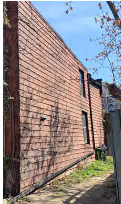
Eastern terrace: south elevation (ERA, April 2022)
