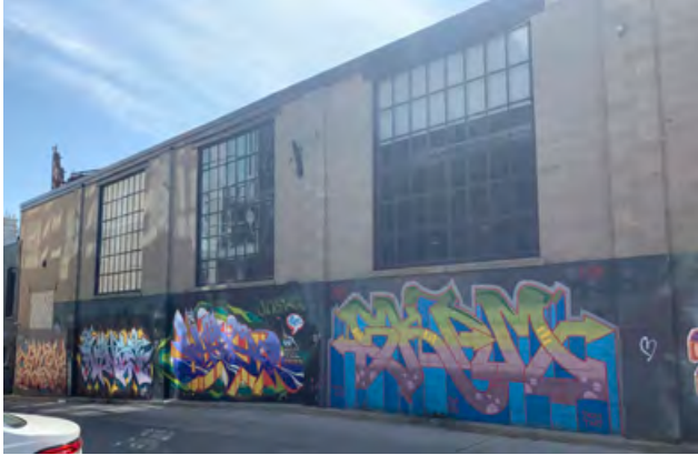
North elevation of 376R Dufferin Street along Milky Way Lane.
