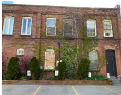
West elevation, three southernmost bays with various eras of window replacements (ERA, 2021).
