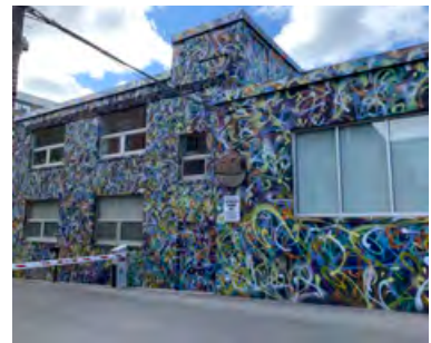
North elevation of the 2-storey building (ERA, 2021).
