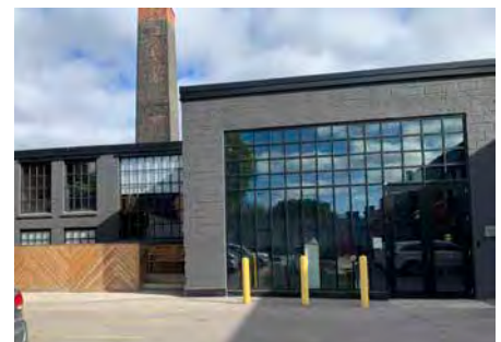
View of south elevation of 376R Dufferin Street from within the courtyard.
