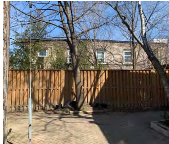
South elevation of 350 Dufferin Street from Melbourne Place.
