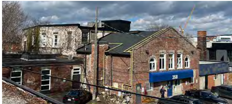
Varied functional building forms, including the mixing building and core oven building at 350 Dufferin Street (more intact) and the foundry building at 358 Dufferin Street (less intact due to loss of gabled roof). The address of the east elevation onto the central courtyard (March, 2022).
