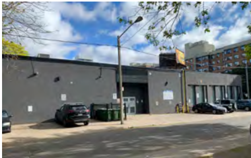
South elevation (ERA, 2021).
