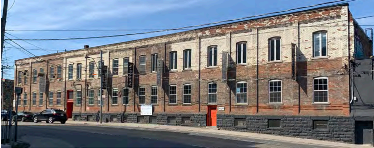
East elevation of 360 Dufferin Street along Dufferin Street.
