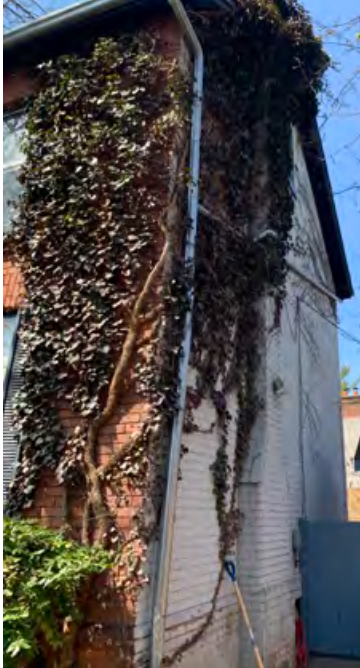
Western terrace: north elevation (ERA, April 2022)
