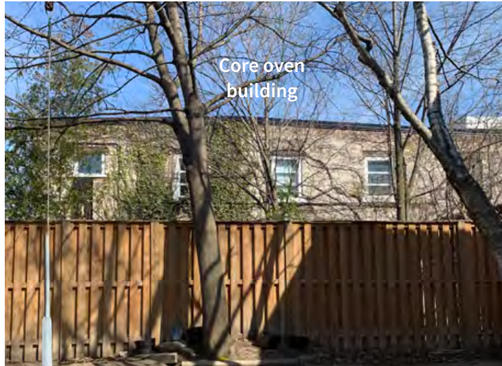
South elevation of 350 Dufferin Street from Melbourne Place.
