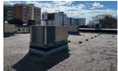
Roof at 340 Dufferin Street (ERA, 2021).
