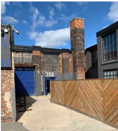
Alternate entrance to 358 Dufferin St. Repairs to chimney are evident (ERA, 2021).
