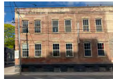
360 Dufferin St. east elevation, 3 southernmost bays and new painted signage (ERA, 2021).
