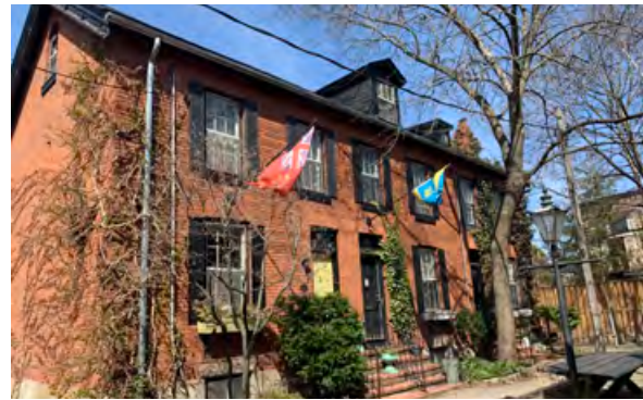
Terraced housing at 1-7 Melbourne Place. Top: 1, 3, 5 and 7 Melbourne Place, Bottom: 2, 4 and 6 Melbourne Place (ERA, April 2022)
