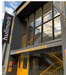
East entrance to 2-storey building (ERA, 2021).
