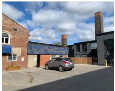
Northwest corner of the courtyard (ERA, 2021)
