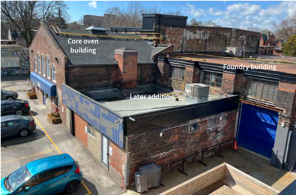
North (and partial east) elevation of 350 (left) and 358 (right) Dufferin Street. Note: March 2022.
