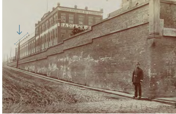
1896 photograph of the Site along Dufferin Street one year after the addition at 360 Dufferin Street was added (indicated with arrow) (City of Toronto Archives; Annotated by ERA).
