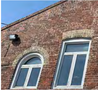
Red brick with contrasting buff brick lintels. Arched and segmentally-arched openings.
