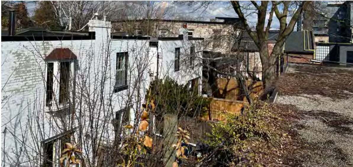
East elevation of 1, 3, 5 and 7 Melbourne Place from the rooftop of 2 Melbourne Avenue (Note: March 2022)
