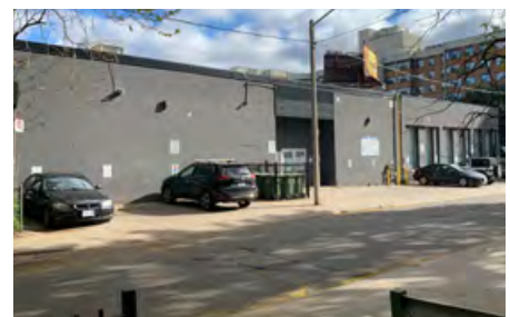
South elevation of 2 Melbourne Avenue and 340 Dufferin Street. Note: May 2021.
