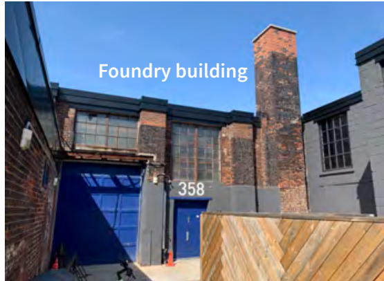
East elevation of 358 Dufferin Street from within the interior courtyard parking area.
