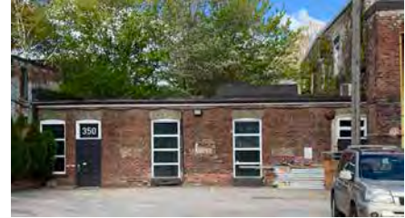
East elevation of the mixing building from the interior courtyard.
