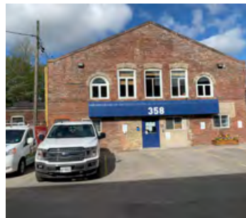
West elevation of 358 Dufferin Street with original windows and doors replaced (ERA, 2021).
