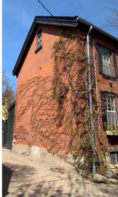
Western terrace: south elevation (ERA, April 2022)
