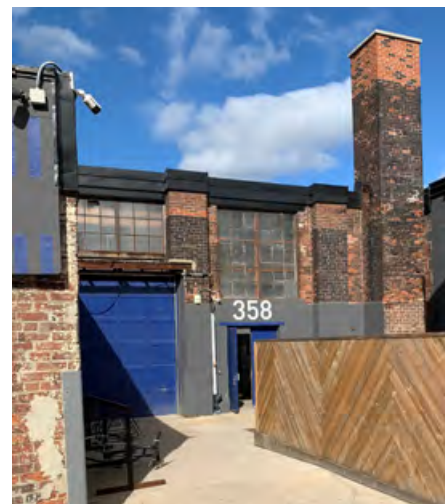
East elevation of the foundry building.
