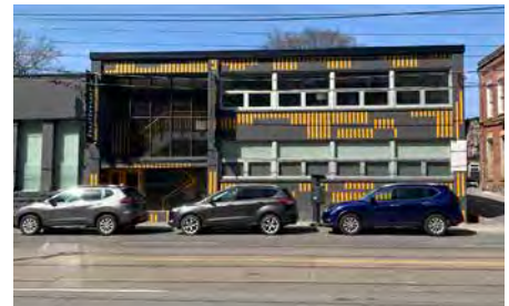
East elevation of 342 Dufferin Street along Dufferin Street.
