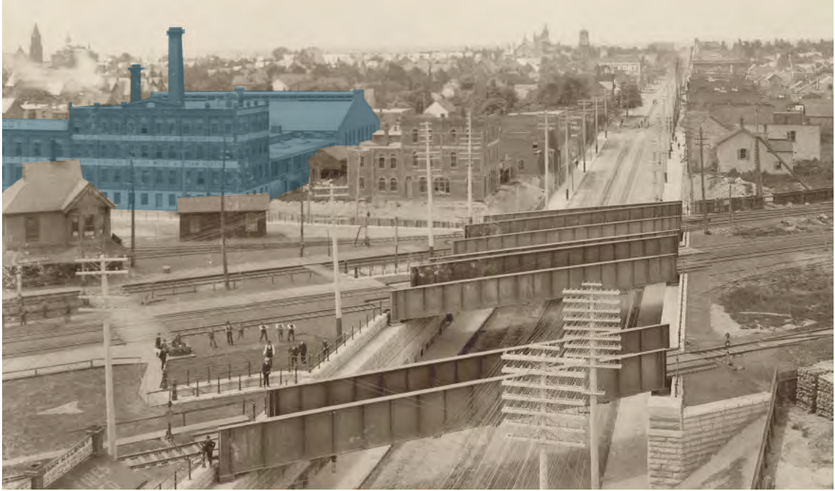
Circa 1898 photograph across Parkdale and the intersection of Queen Street West and Dufferin Street. The newly created rail viaduct is in the foreground. Regrading along the Site's eastern edge on Dufferin Street not only removed the former retaining wall, but also excavated the raised basement of the 3-storey factory building, making it appear as 4-storeys (City of Toronto Archives; Annotated by ERA).
