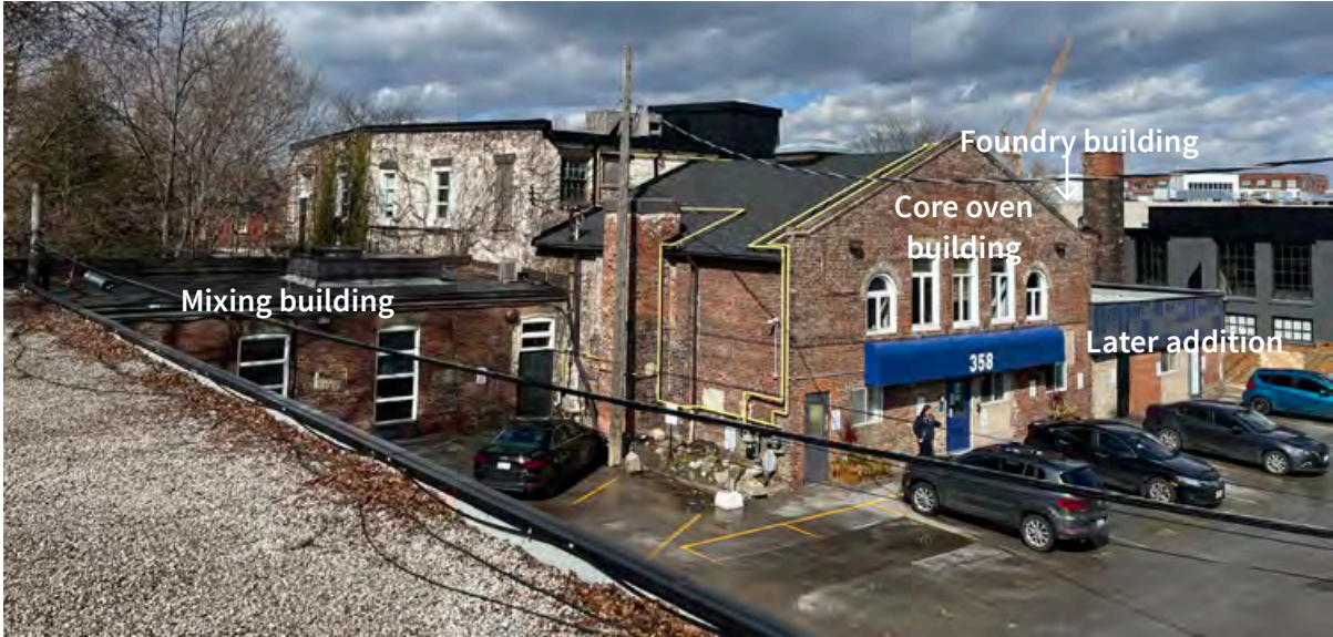
East and south elevations of 350-358 Dufferin Street. Note: March 2022.
