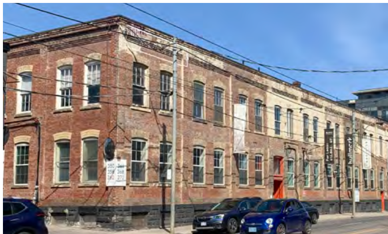
Rectilinear form with flat roof and repetitive bays. Two-storey massing.
