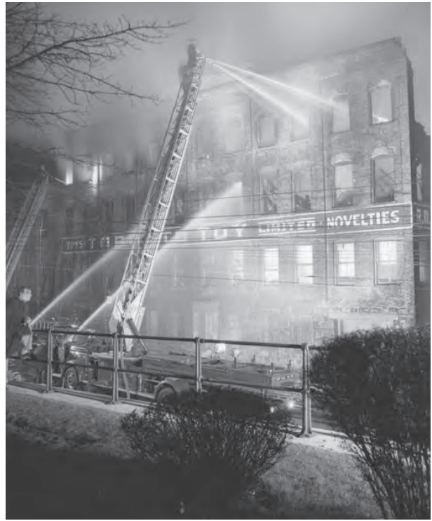
1953 fire that destroyed the top floors of the factory building at 366-370 Dufferin Street. These floors were not rebuilt. (City of Toronto Archives).
