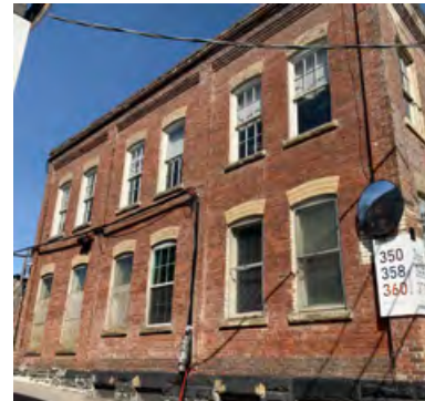
South elevation of 360 Dufferin Street from private east-west driveway.
