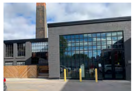
View of south elevation of 376R Dufferin Street from within the courtyard.
