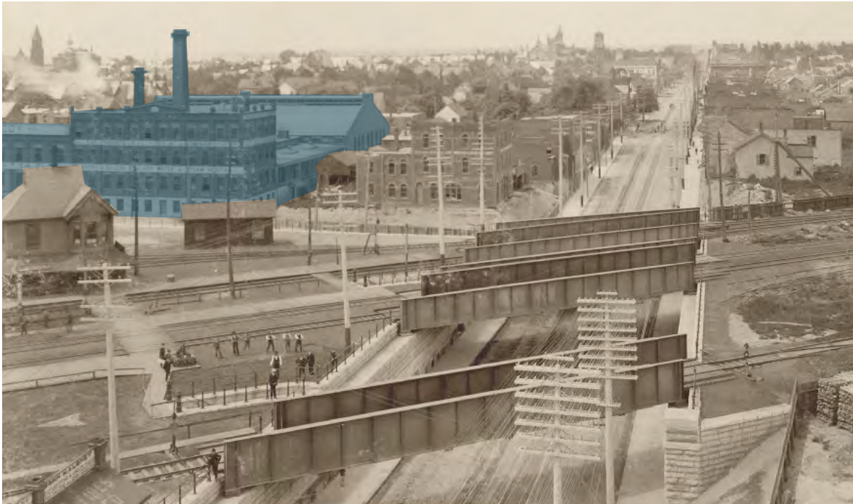
Circa 1898 photograph across Parkdale and the intersection of Queen Street West and Dufferin Street. The newly created rail viaduct is in the foreground. Regrading along the Site's eastern edge on Dufferin Street not only removed the former retaining wall, but also excavated the raised basement of the 3-storey factory building at 366-370 Dufferin Street, making it appear as 4-stores. (City of Toronto Archives; Annotated by ERA).
