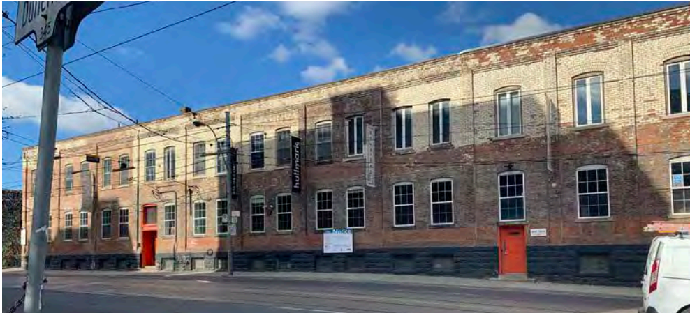
East elevation of 360 Dufferin Street from Dufferin Street (ERA, 2021).
