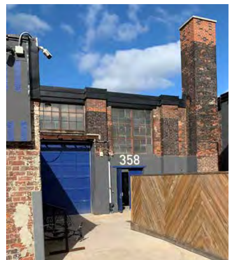
East elevation of the foundry building.
