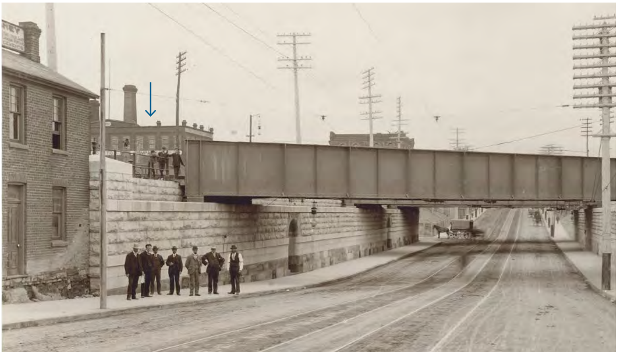
Circa 1898 photograph west along Queen Street West. A large chimney with corbelling (no longer on the Site) can be seen (City of Toronto Archives; Annotated by ERA).
