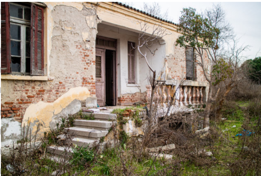
Abandoned building, Thessaloniki and surroundings Benj Herren 2021
