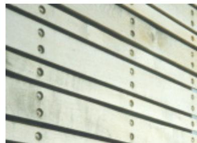
Un-treated timber rainscreens are easy to re-use if bolted.
