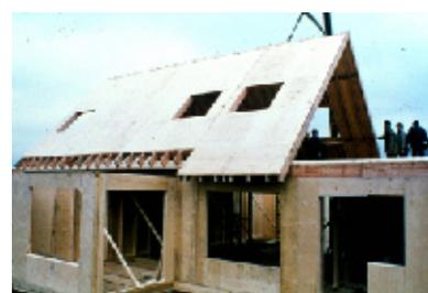
Pre-fabricated composite panelling structure.
