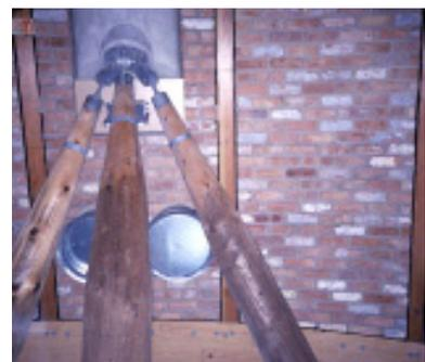
Example of re-used timber telegraph poles as structural members.
