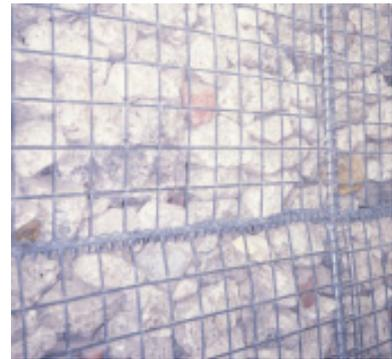
Gabions enable low grade materials to be recycled, but check that wiring will last.
