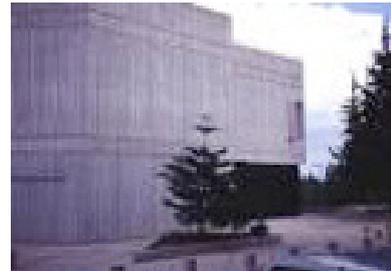
In-situ concrete can be an “immovable construction”, which is hard to deconstruct.
