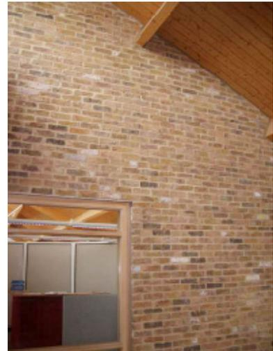
Re-using bricks depends on using soft mortar joints where possible.
