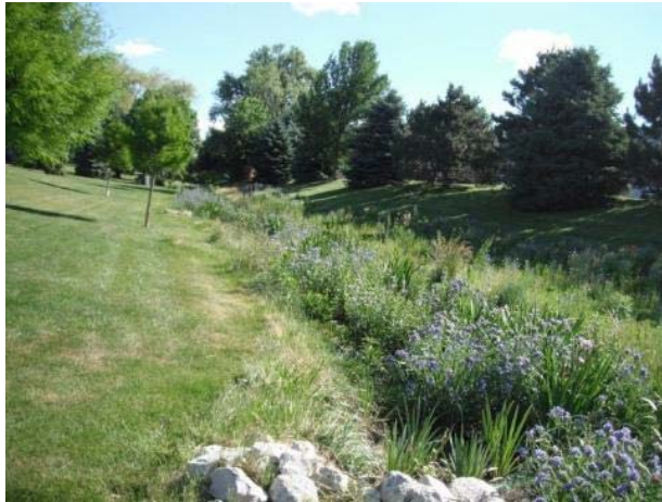
Figure 34: Example of vegetated open swale in Maryland.
