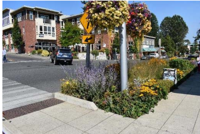
Figure 16: Green Street in Bainbridge, WA that has bioretentions installed into the sidewalk with curb cuts.
