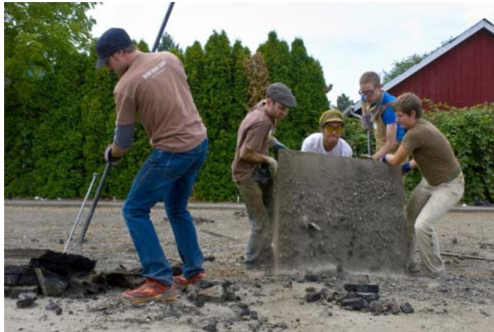
Figure 7: Depave, a non-profit from Seattle, WA organizes volunteer groups to manually remove impervious surfaces.
