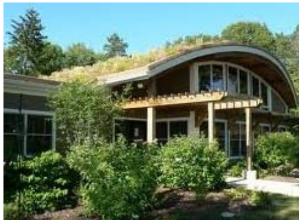
Figure 15: A green roof on top of a nature center in Pennsylvania.
