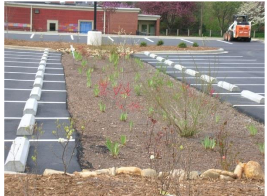
Figure 33 Curb less Traffic Island Bioretention Cell (2005)
