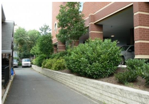
Figure 40 Bioretention Cell in a wall at the Read Building -Falls Church VA
