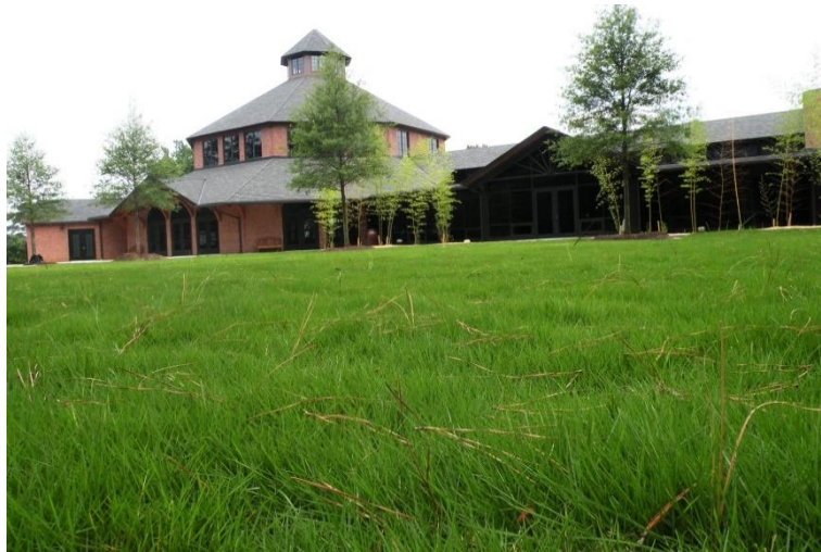
Figure 3 Cape Fear Botanical Gardens –Fayetteville NC- Load Bearing, High Infiltration Stalite Media with Zoysia Turf Overlay.
