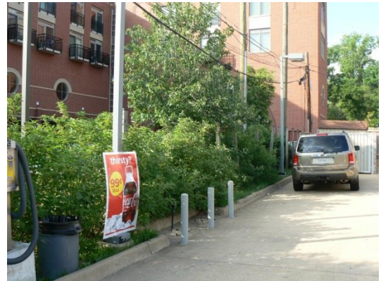
Figure 38 Bioretention Cell between the Read Building and a Gas Station
