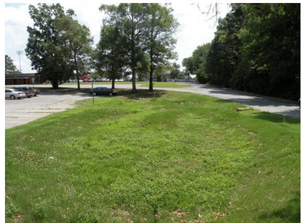
Figure 24 Cell in place (2010)
