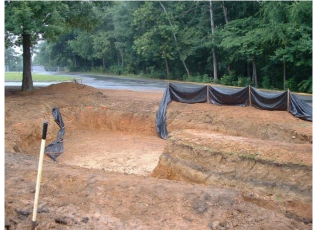
Figure 22 Excavation of two Bioretention cells (2005)
