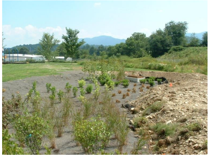
Figure 30 Hazelwood Elementary School - Waynesville, NC (2005)
