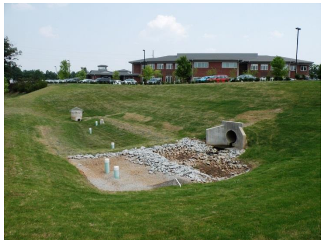
Figure 16 Hospice of Wake County Bioretention Cell with Bermuda Turf Overlay - Raleigh, NC (Summer 2012)
