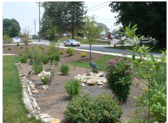
Figure 34 A Roadside Bioretention Transylvania County Public Library - Brevard, NC (2007)
