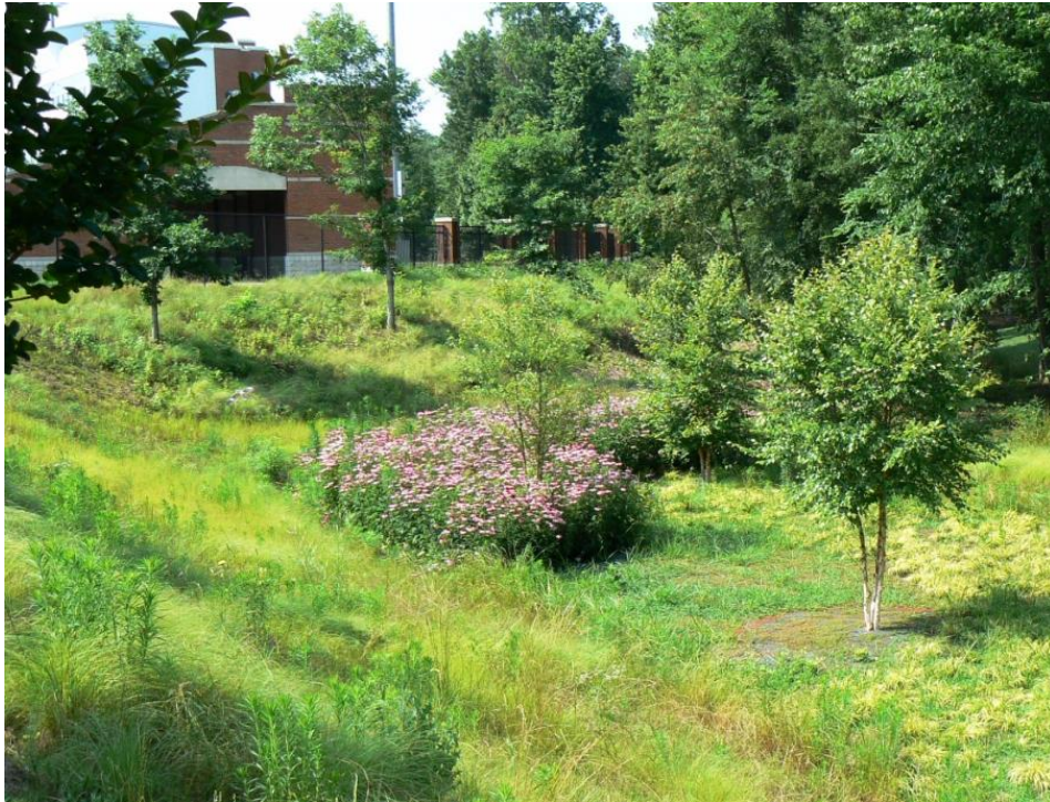
Figure 4 Bioretention Cell at the Alumni Field House - Elon University in Elon, NC (2012)
