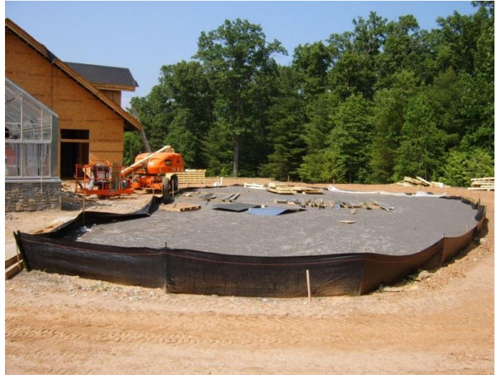
Figure 27 Baker Exhibit Center Event Turf during installation (2008)
