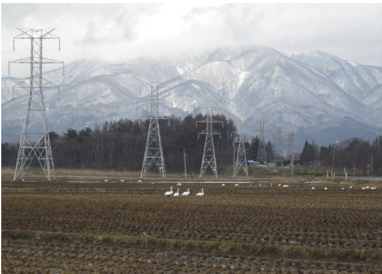
154kV Inawashiro Kyu-kansen transmission line (TEPCO Power Grid)
