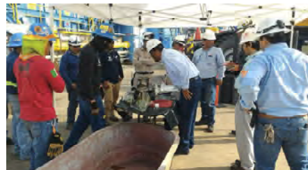
▲ Inspection support (Tuxpan II IPP in Mexico)
