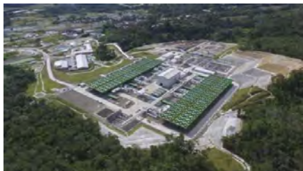
▲ One of the largest geothermal IPPs in the world (Sarulla IPP in Indonesia)
