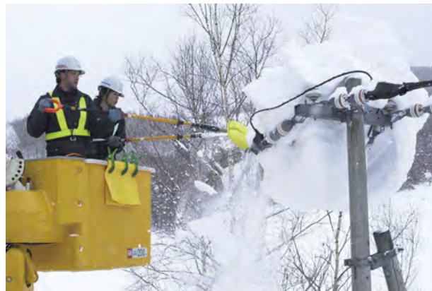
Removing snow from power lines (Hokkaido Electric Power Co.)
