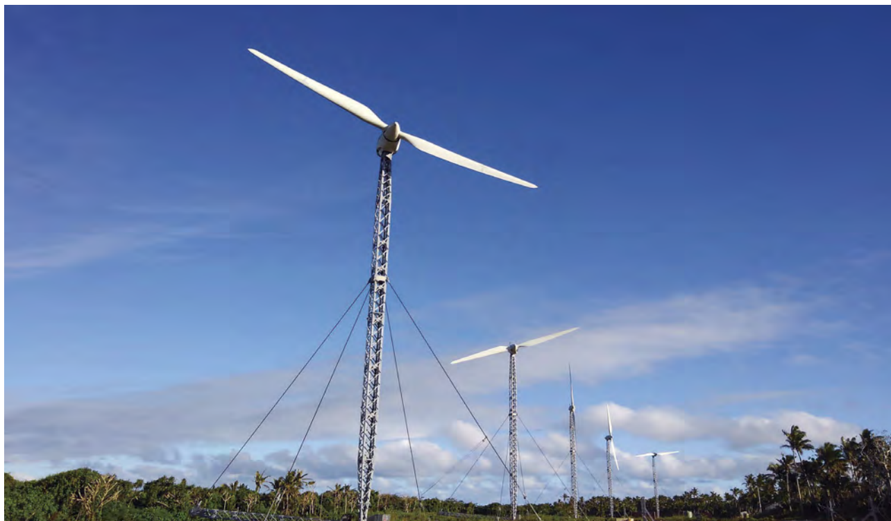
Folding wind turbines being promoted by Okinawa EPco delivered to Tonga (Okinawa Electric Power Co.)
