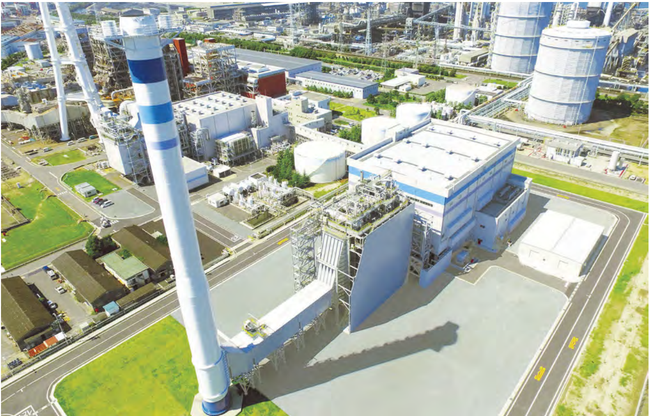
Unit 2 of Sakaide Power Station (Shikoku Electric Power Co.) Reentered service after conversion from oil to LNG-CC in August 2016.
