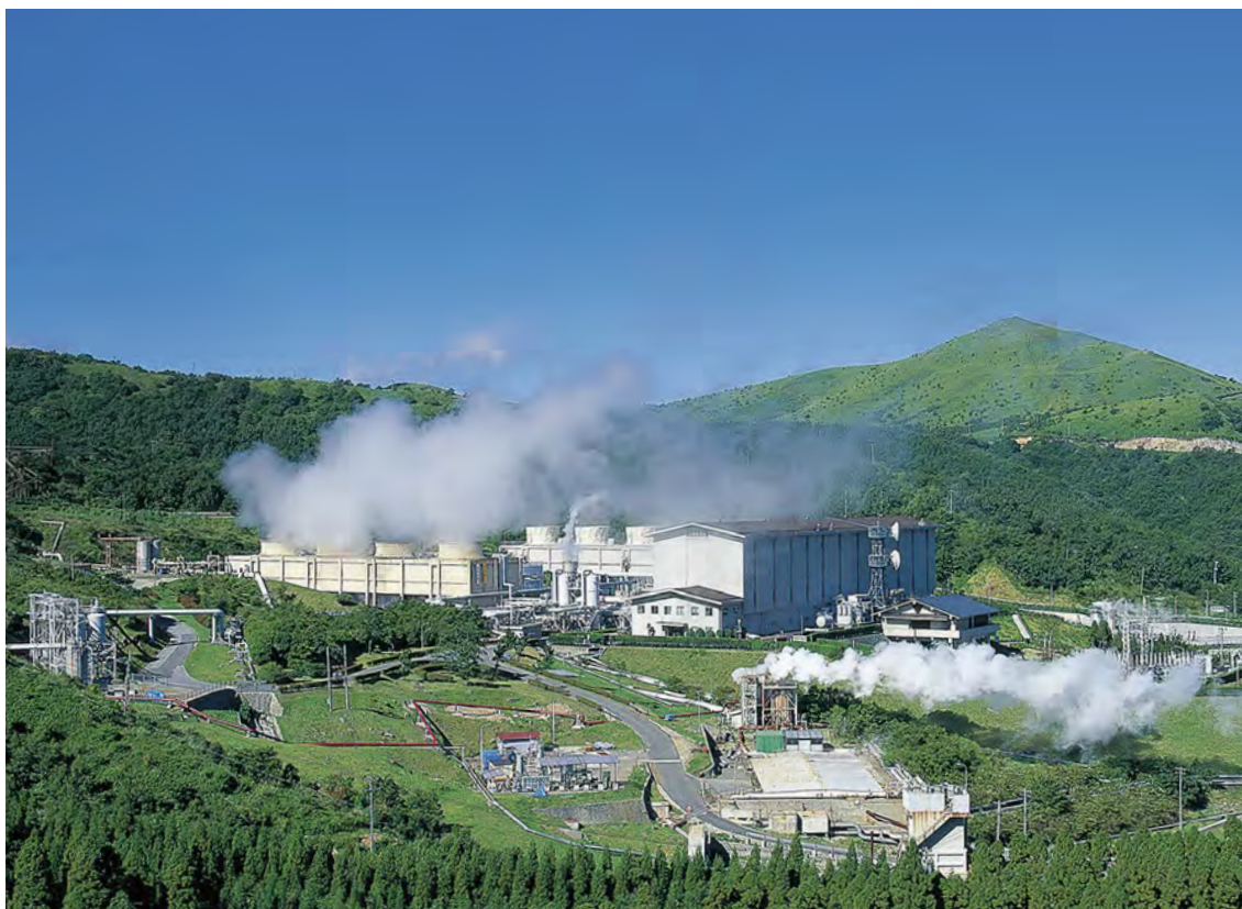
Hatchobaru Geothermal Power Station (Kyushu Electric Power Co.)
