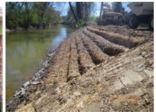
Figure 5. Existing Bank Condition and Example of Geolift Bank Construction with Rock Toe
