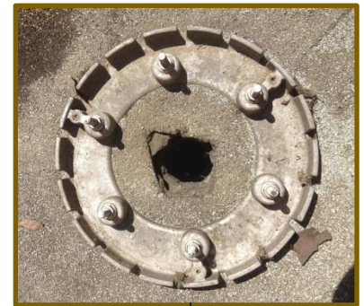
Access and Condition of 3” roof drain before lining
