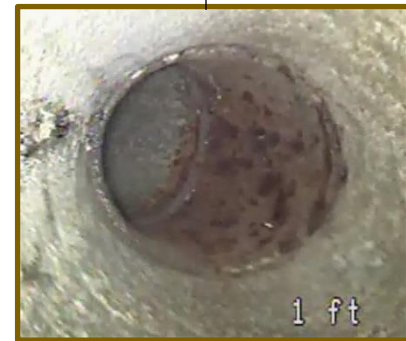
Access and Condition of 3” roof drain before lining
