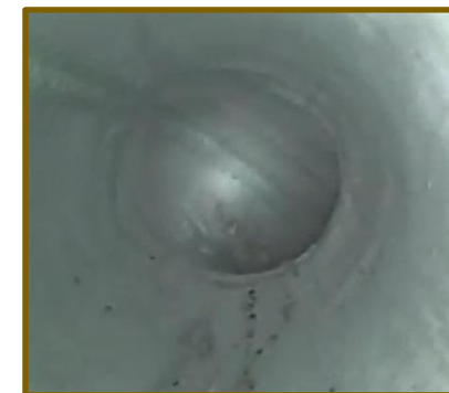
3 inch roof drain after Flow-Liner® installed
