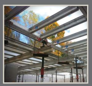
**DROP PANELS**can efficiently be hung from slab framing with our hanger system.
