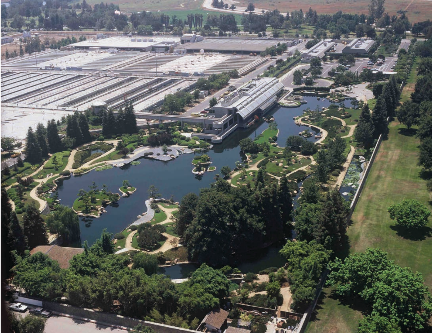
Donald C. Tillman Reclamation Plant.
